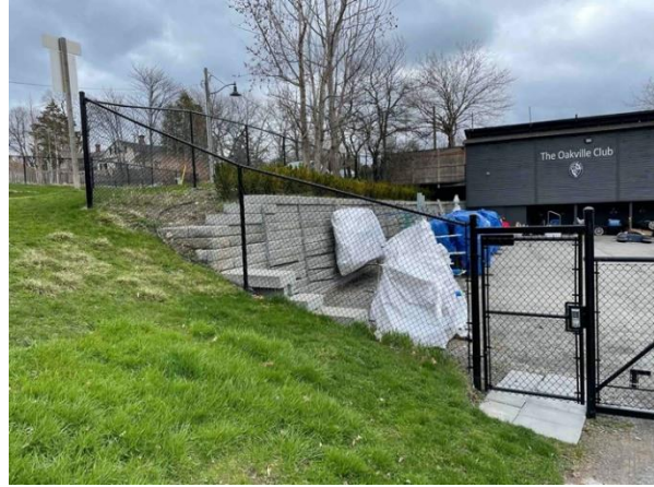
Photo 14 – Retaining wall at The Oakville Club.
