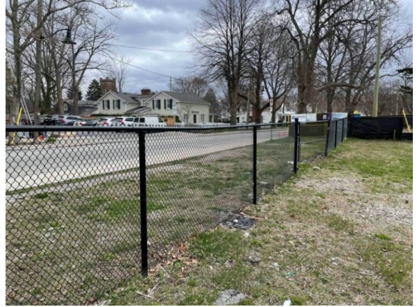
Photo 6 – View along eastern fence at Navy Street, looking south.
