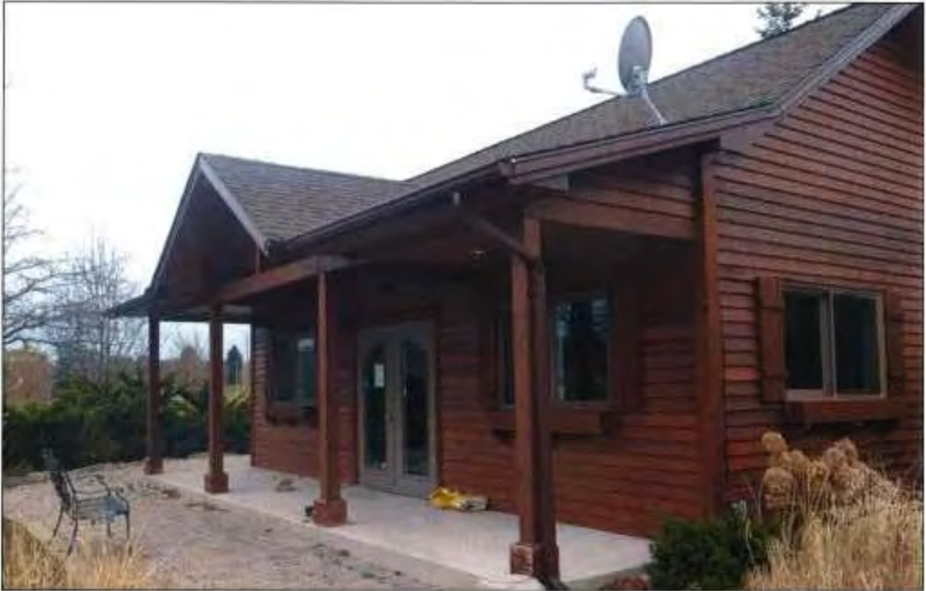
Photograph 12 Front View of the Office Building
