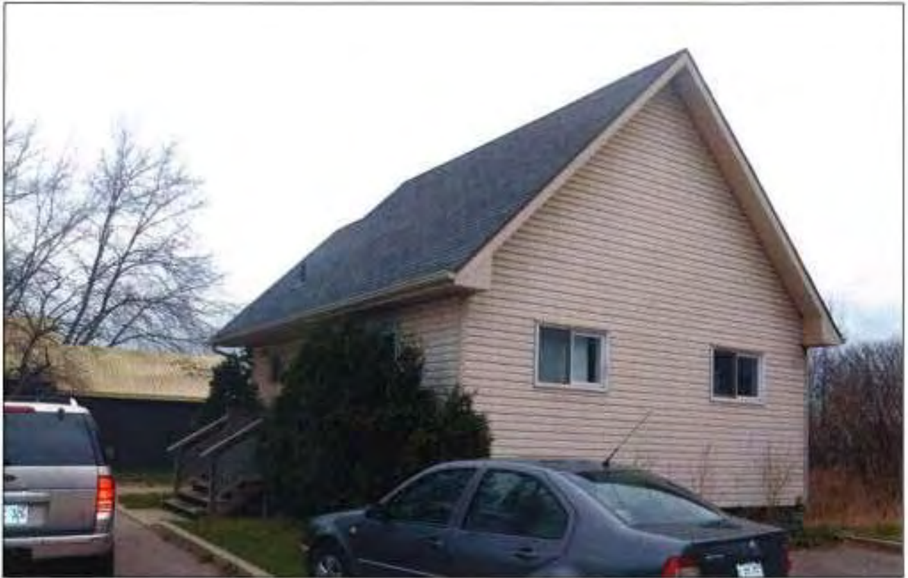
Photograph 16 View of Maintenance Office Building
