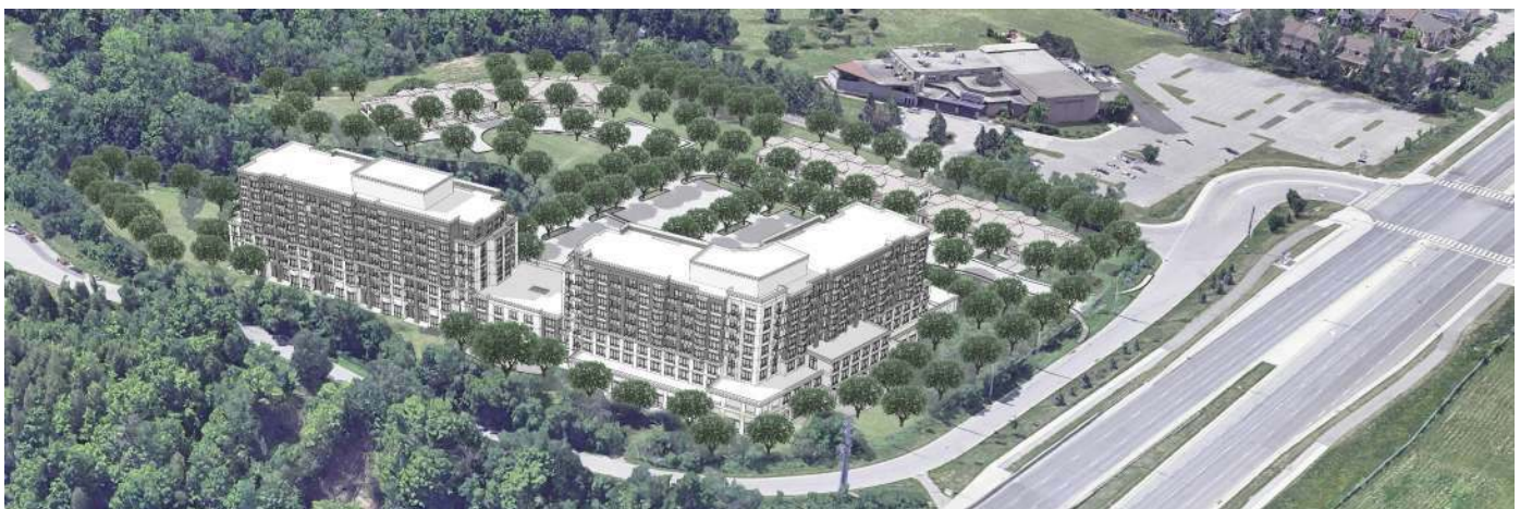
As illustrated, the eight-storey seniors residence has been designed with stepbacks above the podium base. A three-storey podium connects the two towers, which breaks up the overall building mass. The building has been oriented towards surrounding roads including Fourth Line and Dundas Street West and is oriented to provide views of Sixteen Mile Creek.
