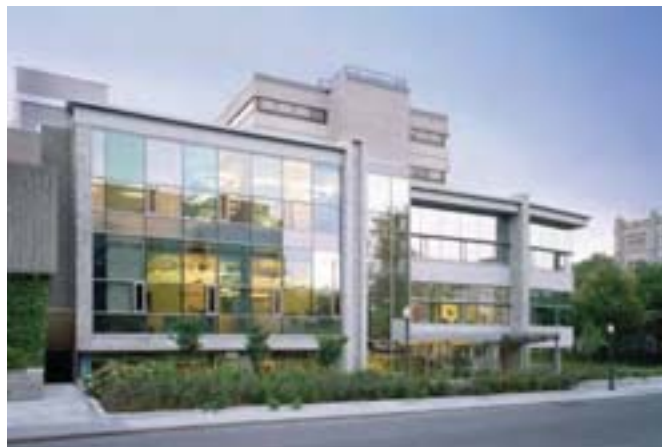
Photo 7.3: Lower scale employment buildings will provide a good transition between the Special Policy Area and the Employment Lands to the North.
