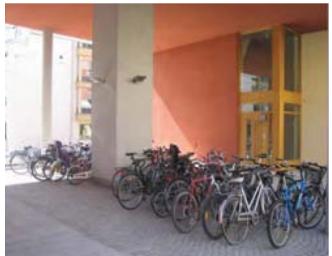
Photos 3.170 & 3.171: Bicycle parking should be convenient and located close to the main entrance of buildings.
