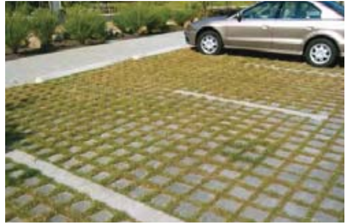
Photo 3.101: On-site stormwater retention areas reduce the requirement for end-of-pipe stormwater infrastructure.
