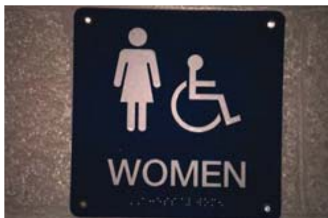
Photo 3.15: Pictorial, written and tactile signage should indicate the location of accessible facilities.
