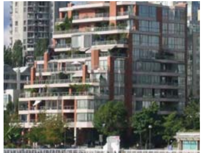
Photo 3.72: Buildings designed with stepbacks can utilize these transitions to create useable outdoor spaces at upper levels, such as patios and terraces with landscaping.
