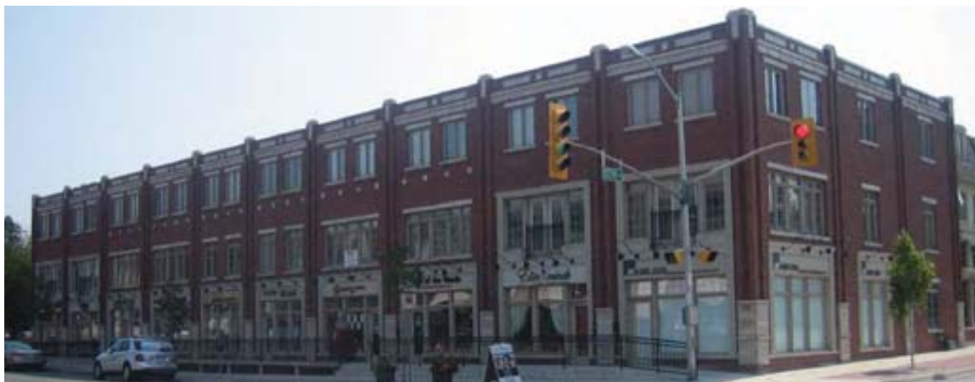
Photo 4.2: Where low-rise buildings on Dundas Street (RR5) are proposed they should preferably have a consistent street wall as a buffer to help mitigate the major transportation role and noise of Dundas Street (RR5).
