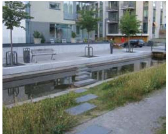
Photo 3.101: On-site stormwater retention areas reduce the requirement for end-of-pipe stormwater infrastructure.
