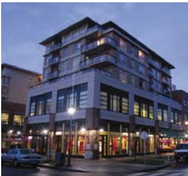
Photo 3.63: The mixed-use nature and tall ground and second floors of this building facilitate flexible tenancies including retail at-grade with office and residential above.
