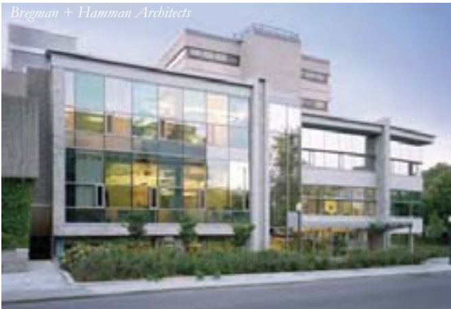
Photo 8.5: Extensive glazing at the street edge and within primary façades promotes quality within the interior spaces and greater integration with outdoor spaces and the street.
