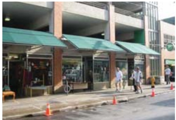
Photo 3.156: Examples of integrated structured parking, note the ground level shops, lack of visible entry point and attention to streetscape.
