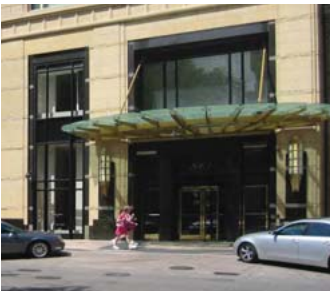
Photo 3.17: A prominent entrance canopy orients visitors, provides weather protection and creates a connection between the building interior and the street.
