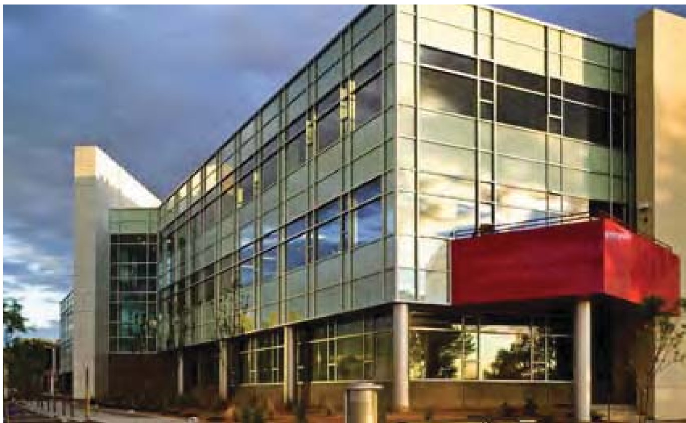
Photo 8.11: Higher design standards are required for employment buildings located on the most highly visible sites.
