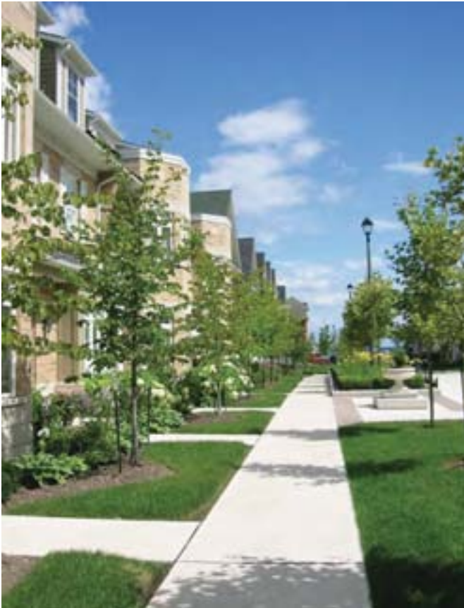
Photo 3.107: Residential sidewalks should be a minimum of 1.5 metres wide.
