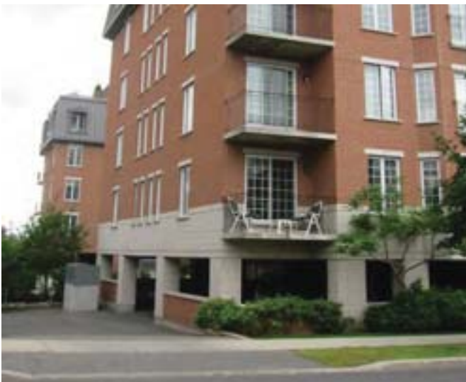
Photo 3.166: The side yard parking garage entrance minimizes its visibility from the street.
