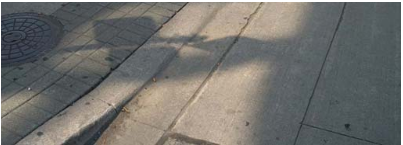
Photo 3.115: Curb ramps should be provided at all intersections. Textured paving also assists those with visual impairments.
