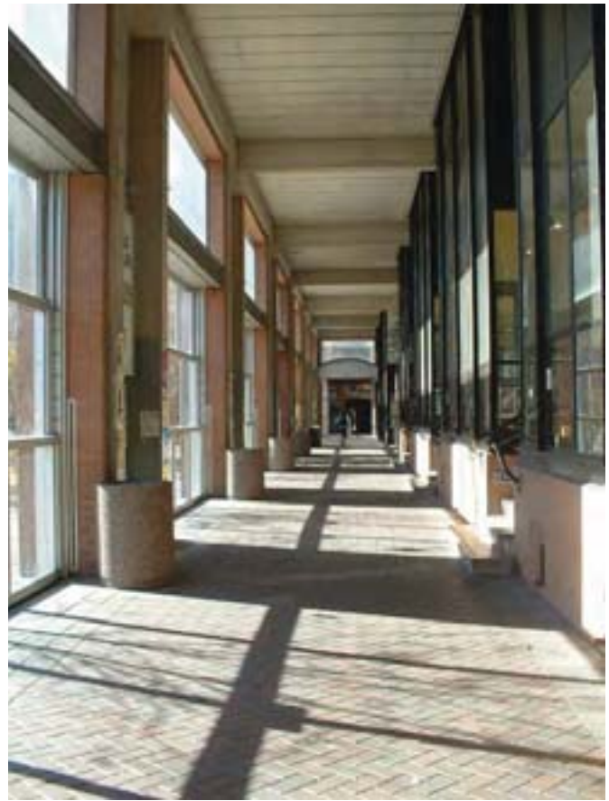
Photo 3.29: Convertible colonnades provide climate protection in winter and shaded breezeways in warmer seasons.
