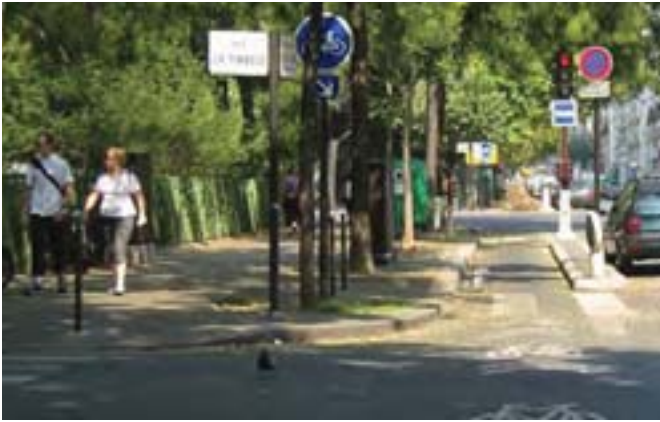
Photo 3.104: This cross section includes sidewalks, trees, cycling lanes, parking and traffic lanes.
