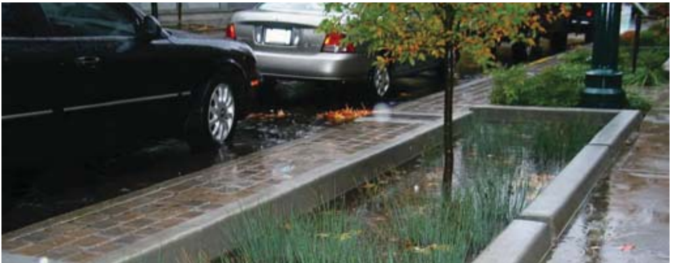
Photos 3.102 & 3.103: Bioswales in naturalized landscapes can help reduce the size of stormwater management ponds.
