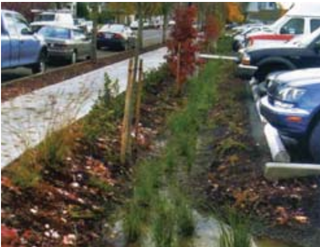
Photo 3.159: Permeable paving, bioswales (as illustrated in this photo) and other features to manage stormwater on-site may be considered, where appropriate.
