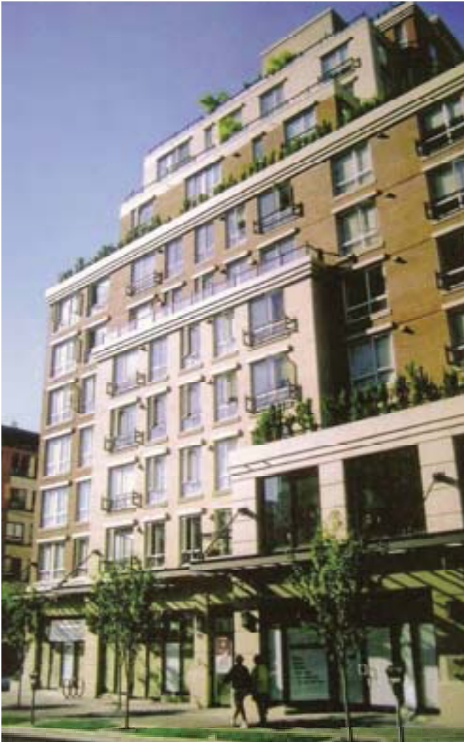
Photo 3.16: Building articulation is used to express the buildings main components: base, middle and top.
