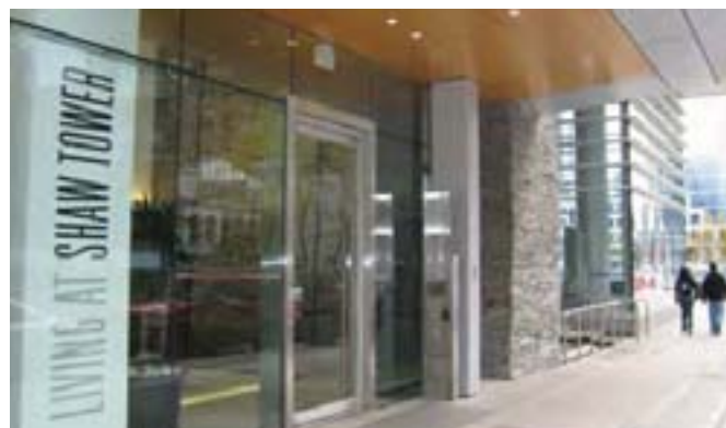
Photo 3.18: Extensive glazing used on the ground floor of this building creates a strong connection between the building lobby and the street.
