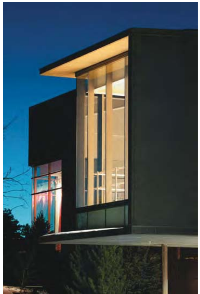
Photos 3.34 & 3.35: The design of outside storage and loading areas should be integrated into the overall building and site design and be constructed of durable high quality materials. The photo above shows a wood screen enclosure and the photo below recesses the storage area under a projecting building element.
