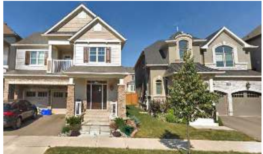
Fig. 6.3.2c - Image example a variety of single detached homes on Carding Mill Trail, south of Argo West Morrison Creek.
