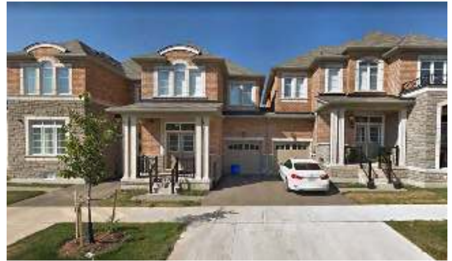
Fig. 6.2.3 - Existing street townhouses located on Carding Mill Trail, south of Argo West Morrison Creek.
