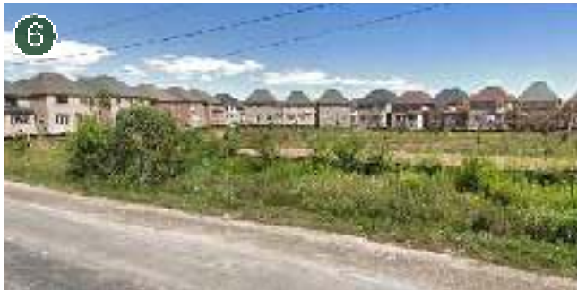
Existing single detached houses under construction backing onto NHS channel along east side of Sixth Line, south east of the Argo West Morrison Creek subject lands.
