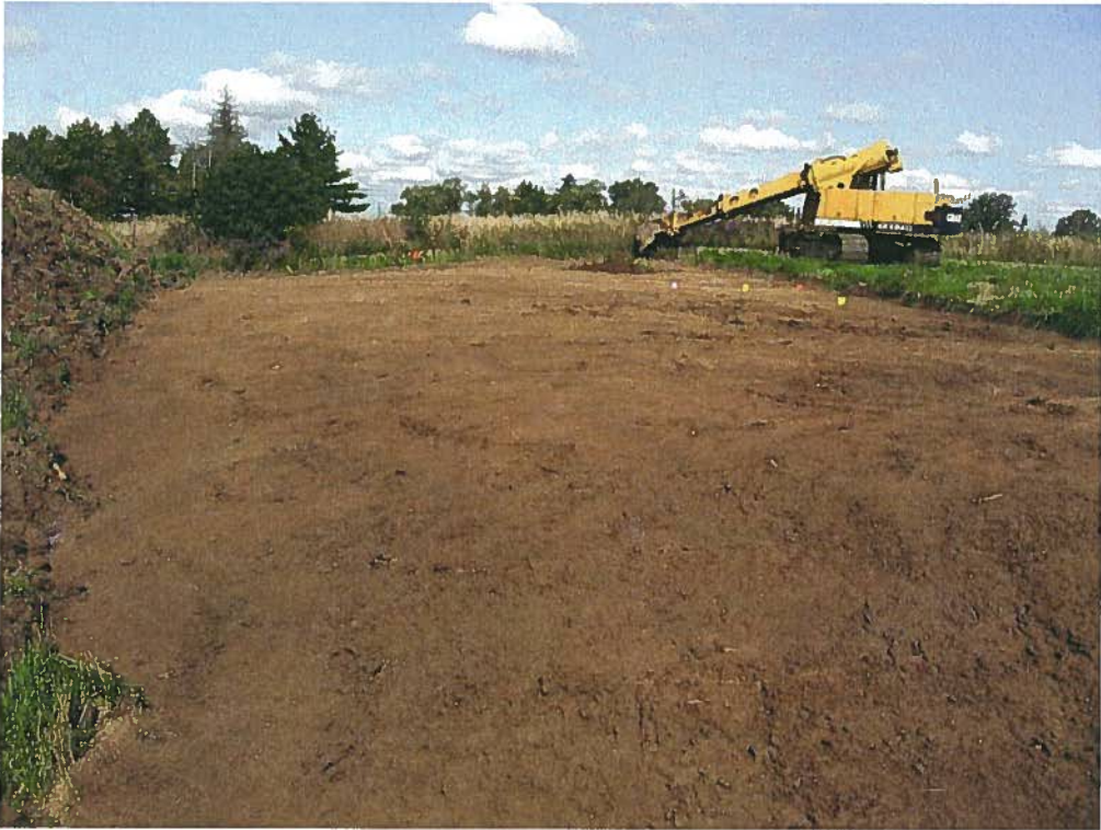
Plate 4: Stage 4 mechanical stripping, looking north.
