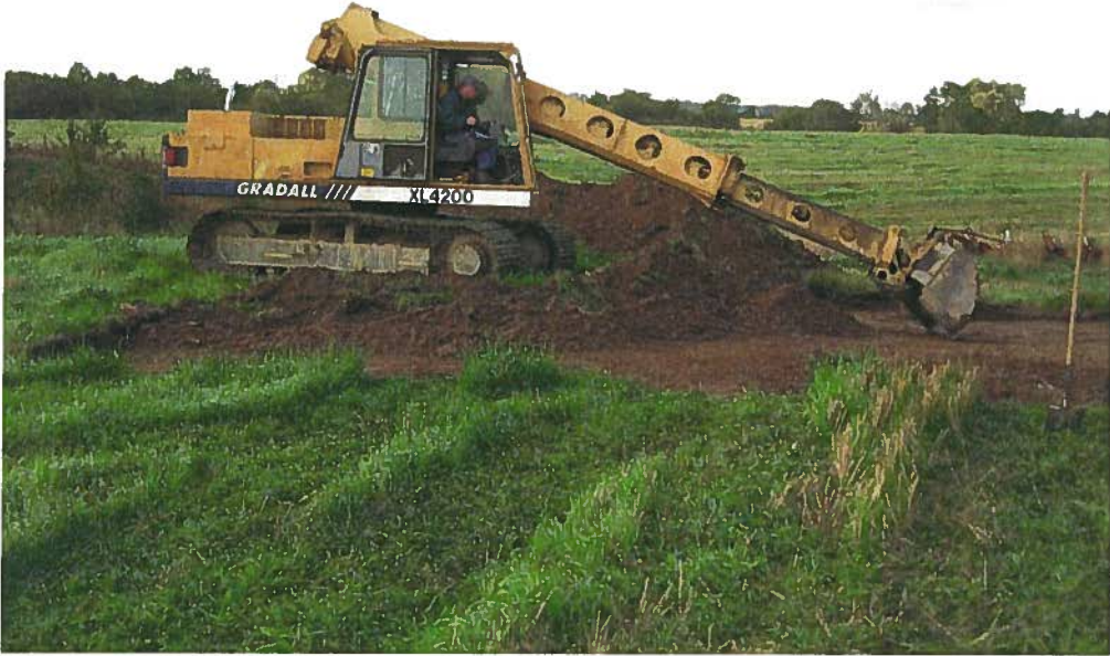
Plate 3: Stage 4 mechanical stripping, looking south.
