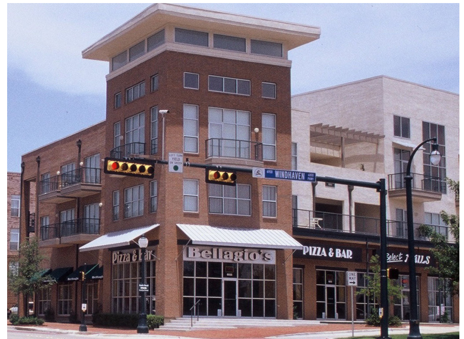
Fig. 5.2.1b - Image examples of mixed use built form, including commercial, retail and residential. Prominent building massing and architectural treatment should be provided at the street edge
