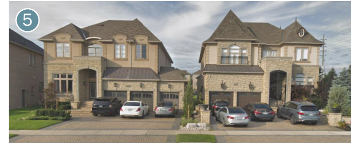
Fig. 2.2d - Single detached homes on Meadowridge Drive, south of the subject lands and Dundas Street W.
