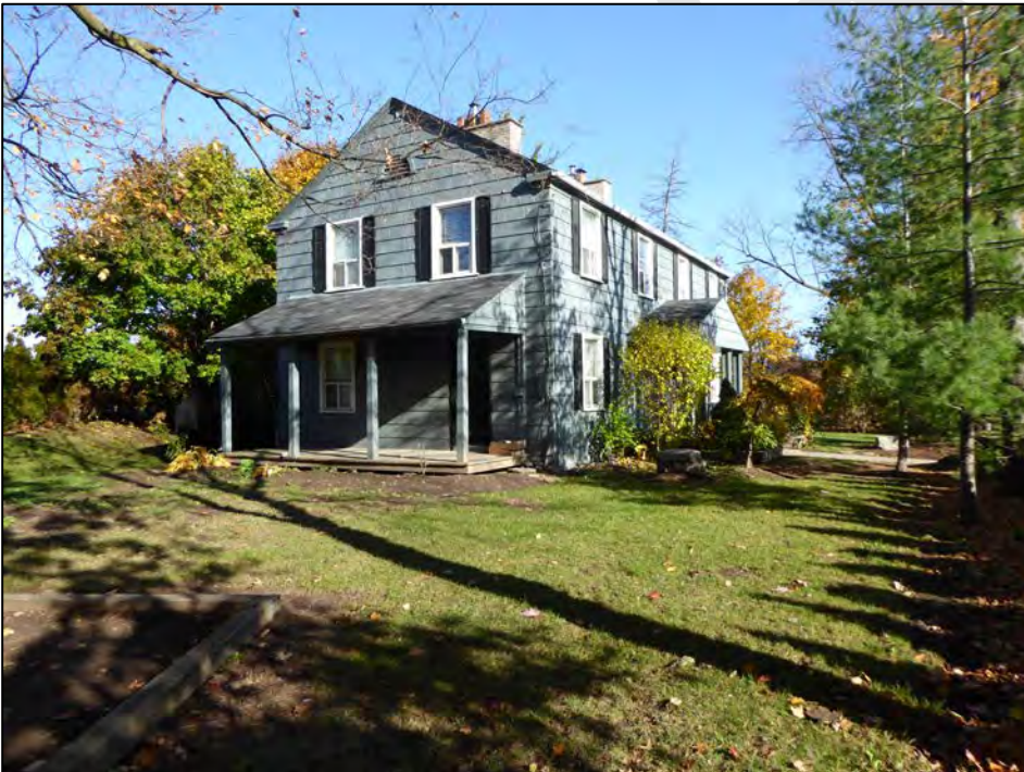
Figure 26: Circa 1937 Staff House, west elevation (JH 2016).
