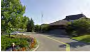
10/ The entrance sequence culminates at the Club House forecourt with a terminal view of the entrance staircase.
