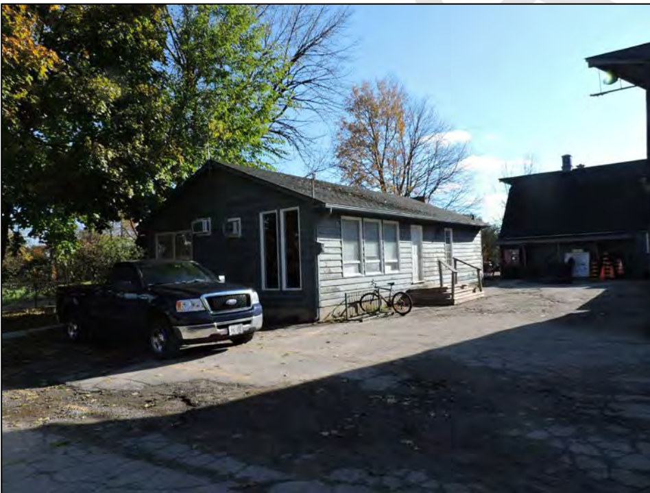
Figure 31: Office building and shed east of stables (AB 2016).
