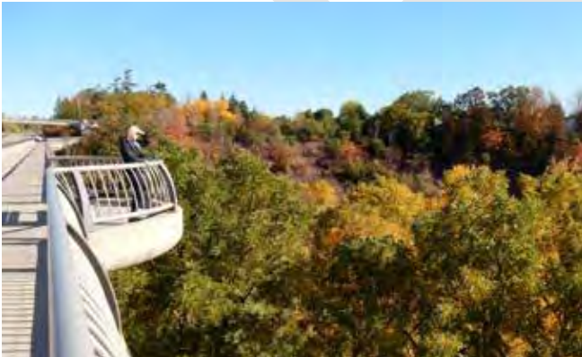
Pedestrian walkways and viewing belvederes incorporated into the Smith Triller Viaduct provide unique viewing experiences over the Glen Abbey and the Sixteen Mile Creek Ravine.
