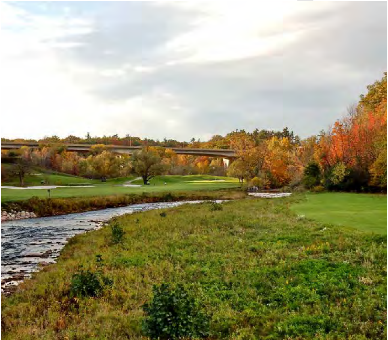
The view northwest along the valley are framed by the valley edges and punctuated by the viaduct, meandering creek and ravine backdrop.
