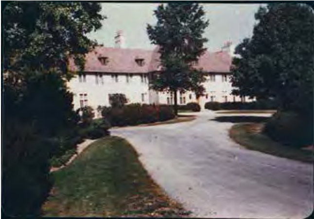
C.2 View of the entrance driveway and turning circle at the house main entrance (circa 1970's)
