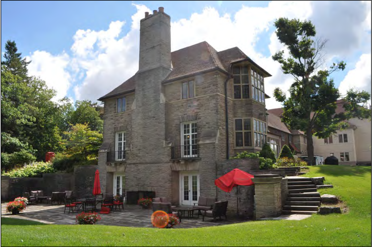
Figure 24: RayDor estate house, basement-level patio at east end of the building giving the appearance of being three-and-a-half storeys (CU 2015).
