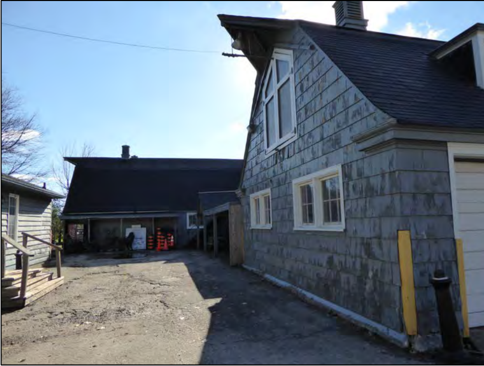
Figure 30: Sheds and office building east of stables (JH 2016).
