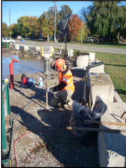
Photograph 1 – Drilling MW-401
