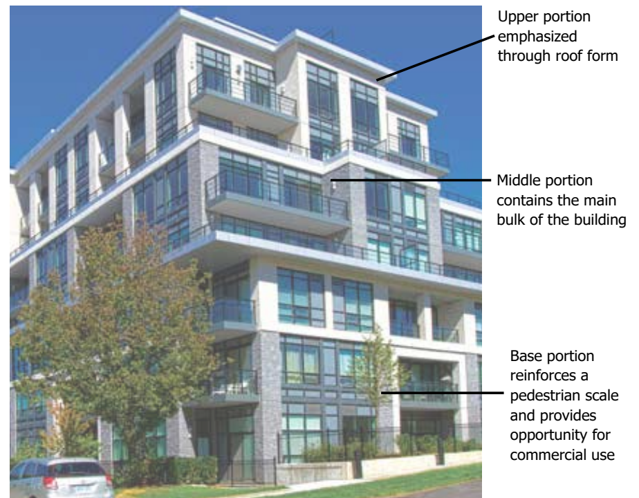
Fig. 6.6.4c - Apartment Buildings should be designed to Establish Distinct Base, Middle and Upper Portions
