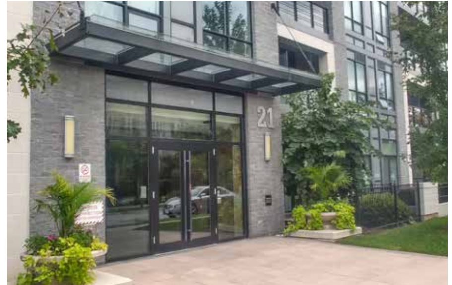
Fig. 6.6.4b - Main Entrances should be Designed as Focal Points for the Mid-Rise Buildings
