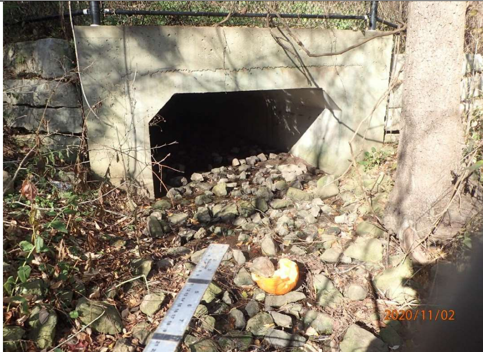
Flows exited the culvert south of Glenayr Gate into a stone treatment. No scour was noted downstream of the outlet.
