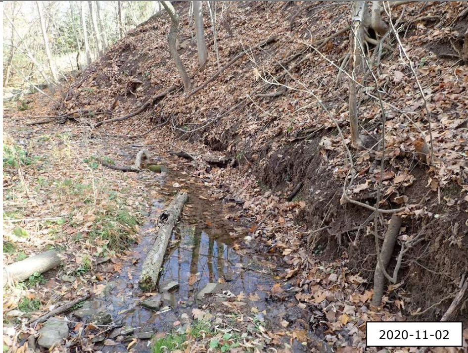
Several instances of valley wall contact and erosion were noted in Reach GC-3 .
