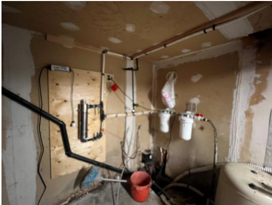
Picture 42: View of the Sump pump and well water treatment station, southwest of Basement.
