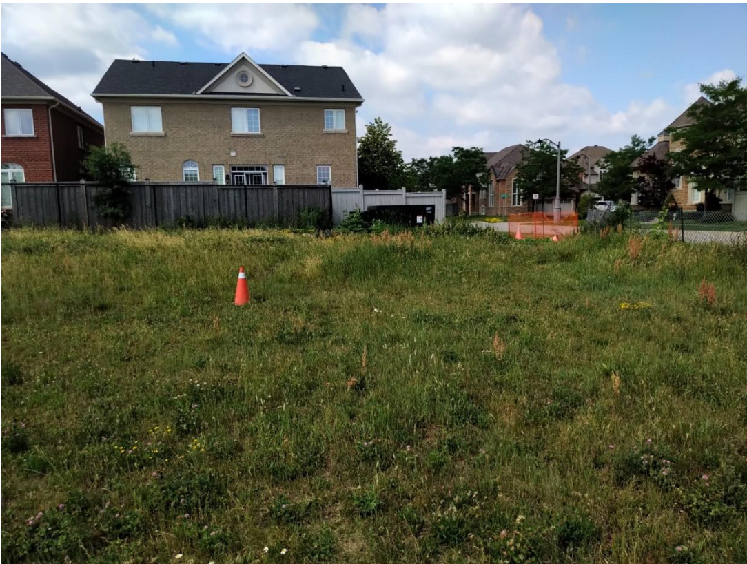
Photograph No. 8 – View of the transformer in the northwest corner of the Site.
