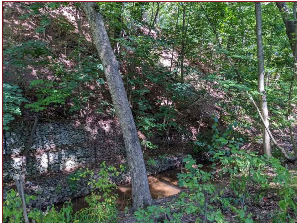
Image 40: Stacked Gabion Baskets at the Base of Steep Slope
