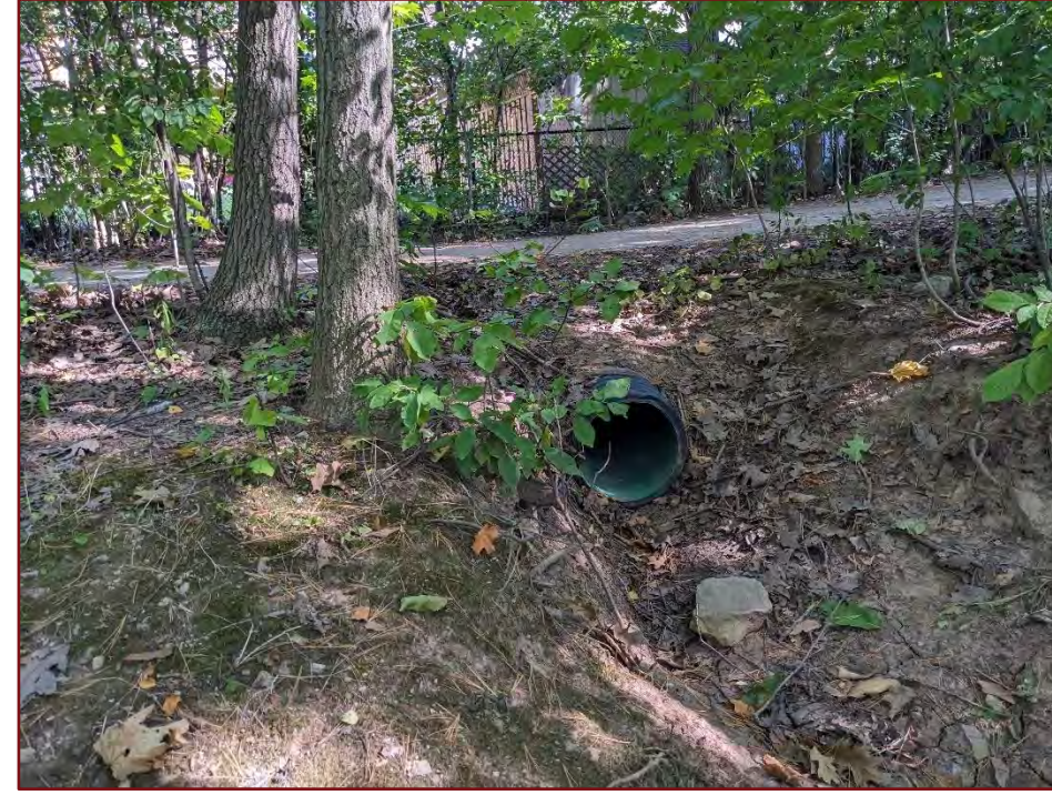
Image 11: Drainage Running Under Trail
