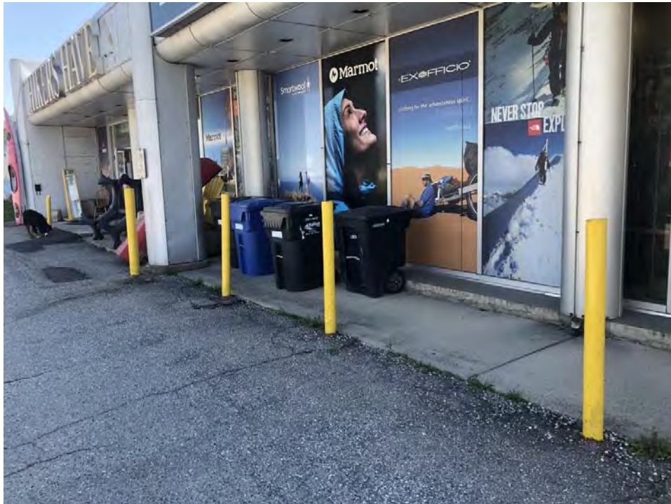
Photo 5: Garbage and recycling bins located on the northern portion of the Site building.
