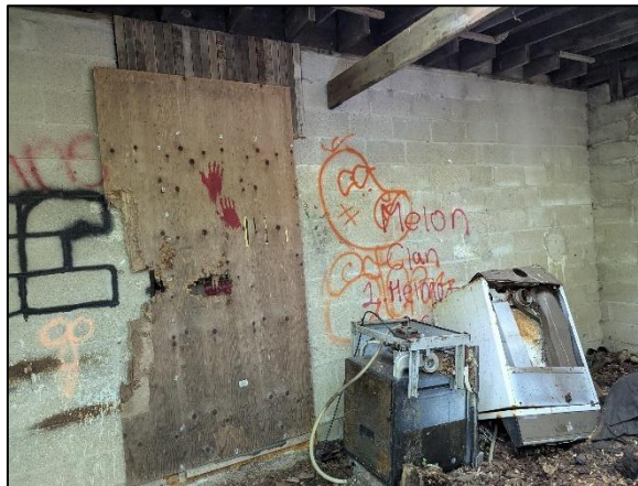
Photograph 23: Concrete Block Wall on East Side of Building
