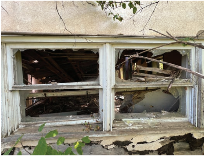
Enlarged window opening at the principal (west) elevation (ERA, 2025).
