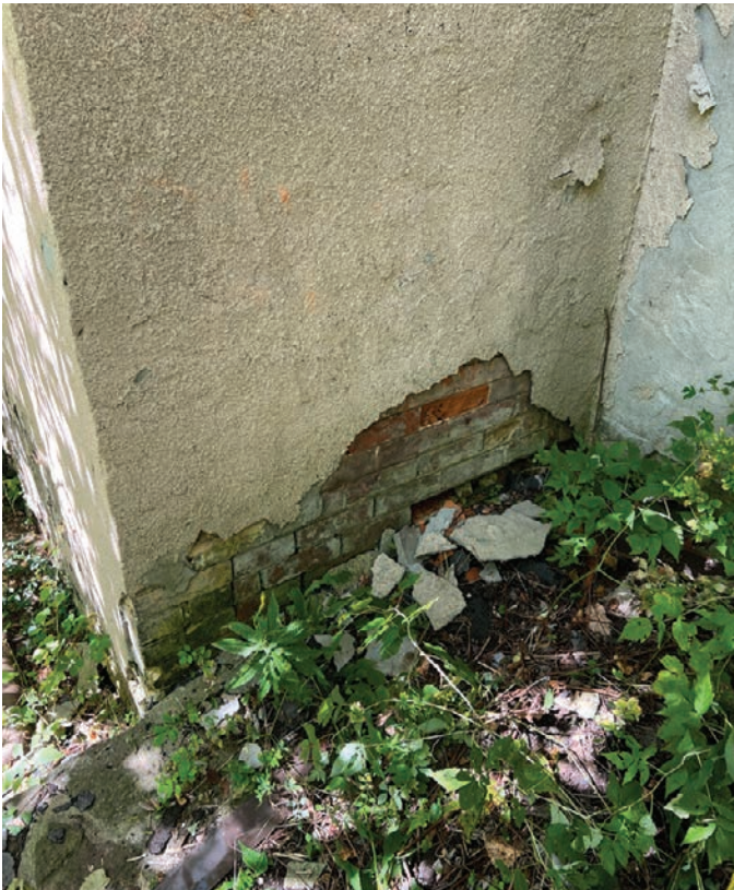
Evidence of masonry underneath the stucco at the original portion of the building. Note the presence of both red and buff brick, suggesting possible buff brick quoining (ERA, 2025).
