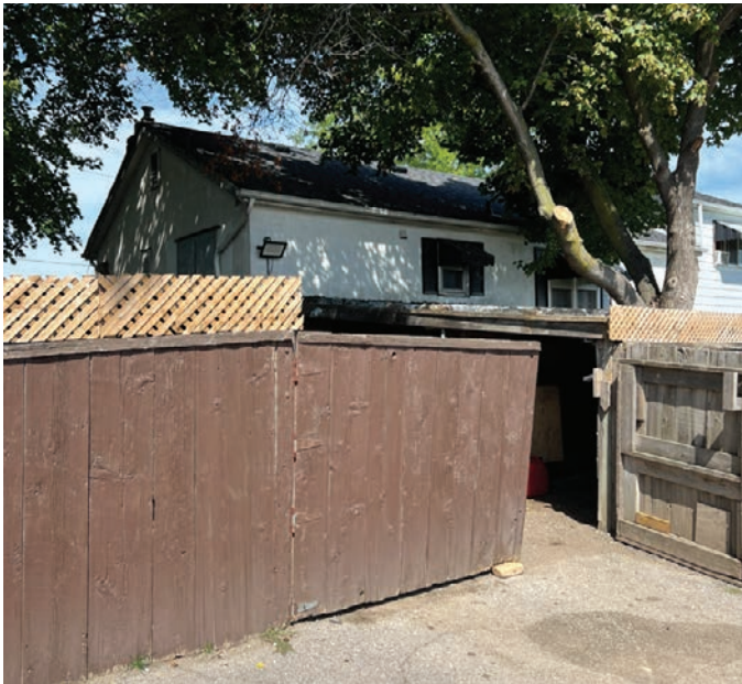
Storage shed at the southeast corner of the building (ERA, 2025).
