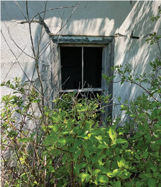
Window opening at the principal (west) elevation (ERA, 2025).
