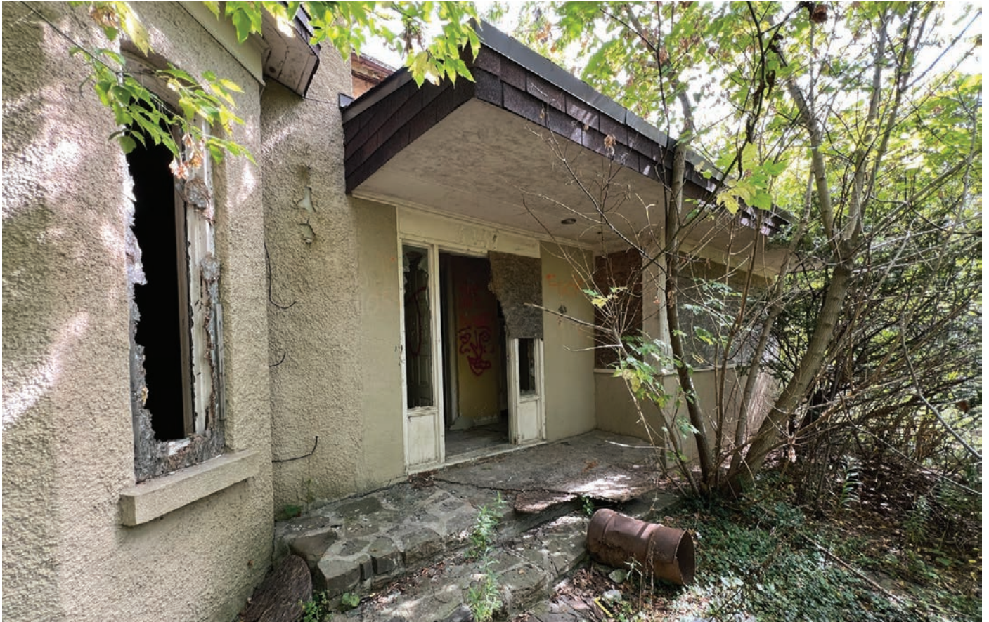
Portion of the principal (west) elevation and main entrance (ERA, 2025).
