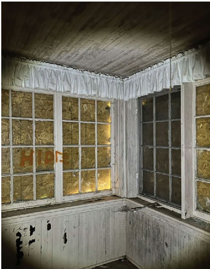
Enclosed sunroom on the ground floor (ERA, 2025).
