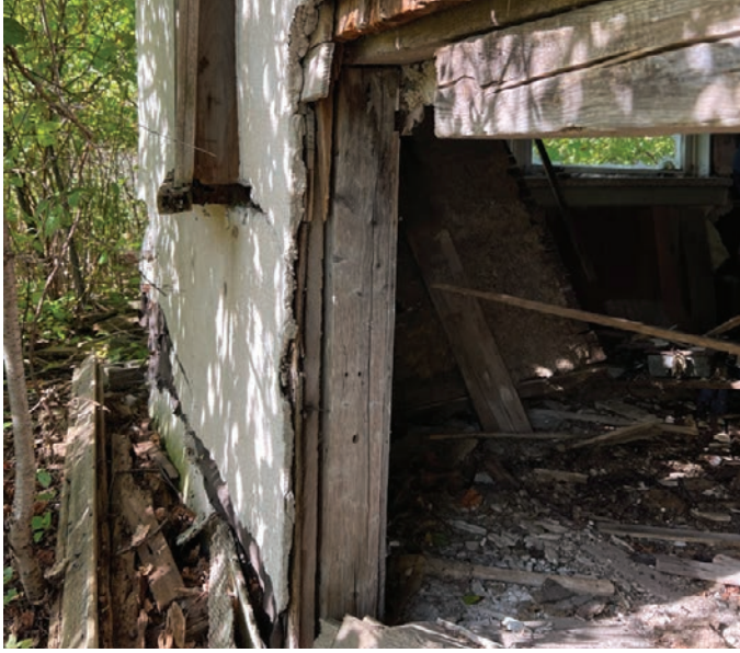
Large opening on the south elevation where a fireplace would likely have been located (ERA, 2025).
