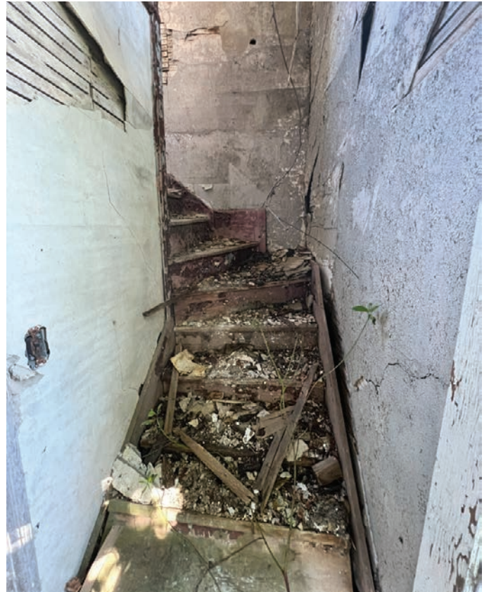
Stairs to second storey (ERA, 2025).
