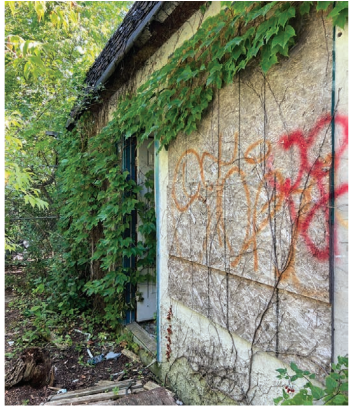
Looking towards the exterior entrance to the rear one-storey addition (ERA, 2025).
