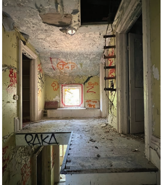
Looking towards the three rooms on the second floor. Note the ladder to the attic (ERA, 2025).
