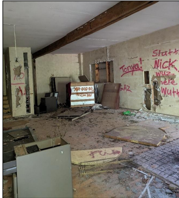
Photograph 20: Built-up Roof Beam in North Addition
