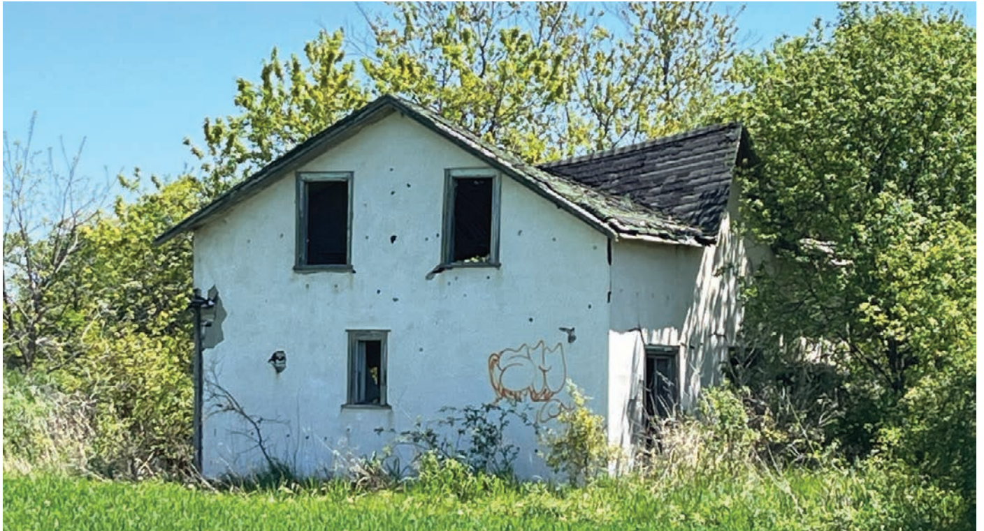
Principal (west) and side (north) elevations of the circa 1840s building at 340 Burnhamthorpe Road (ERA, 2025).
