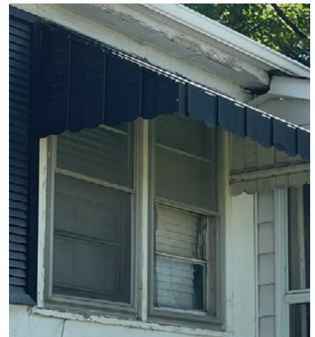
Metal windows in fair condition (ERA, 2025).
