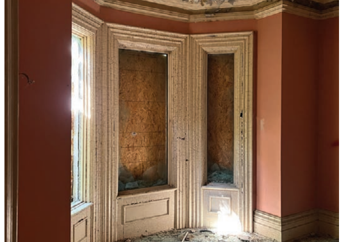
Window surrounds in fair condition (ERA, 2025).
