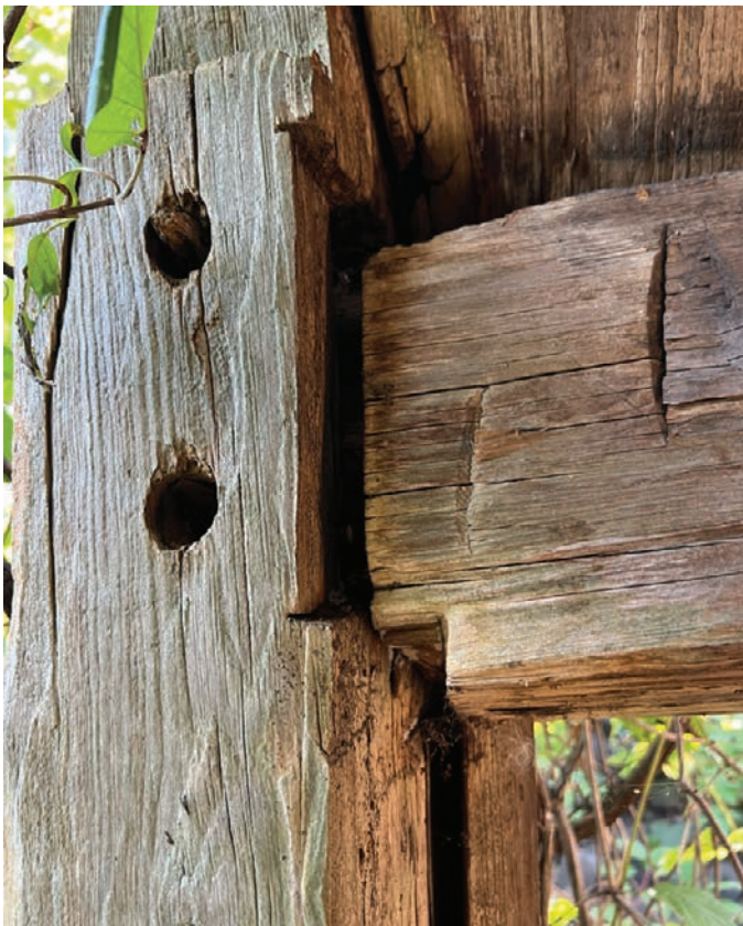
Close-up photo of the mortise-and-tenon joinery at the exterior walls, with wooden dowels connecting the post and beam (ERA, 2025).
