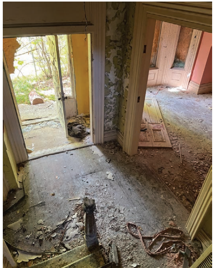
Looking down into the hallway on the ground floor from the staircase (ERA, 2025).
