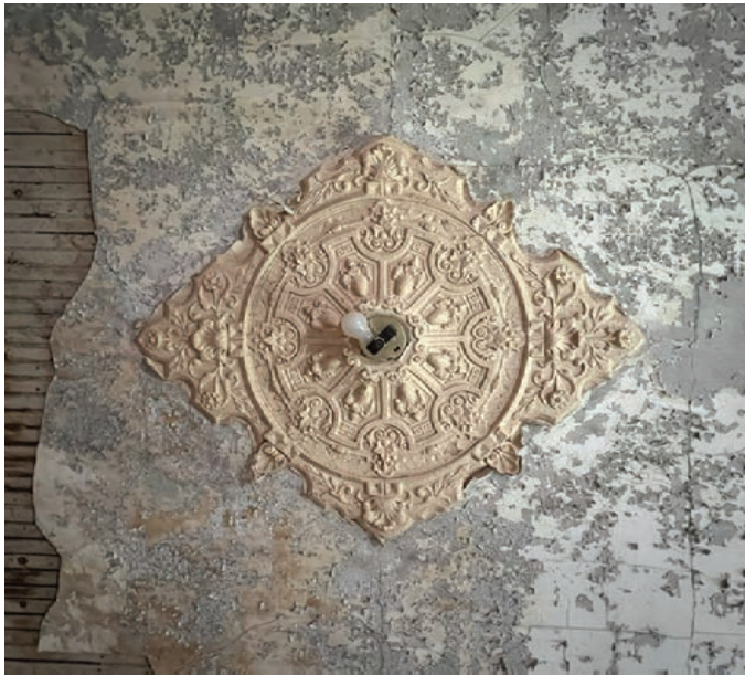
Ceiling medallion on the ground floor (ERA, 2025).
