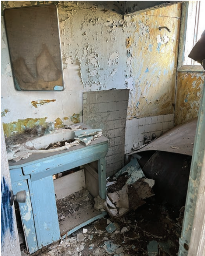
Looking into bathroom on ground floor (ERA, 2025).
