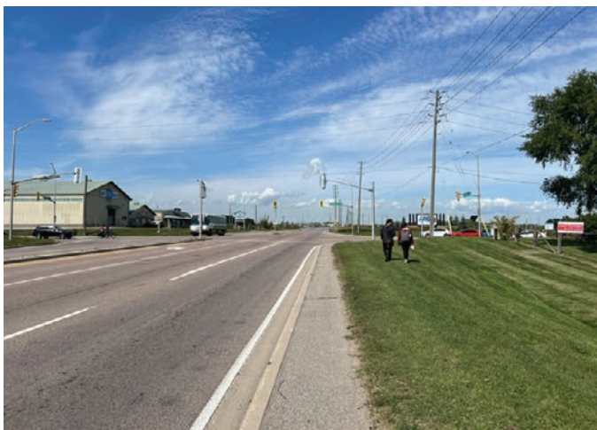
Looking north along Trafalgar Road towards the intersection of Trafalgar and Burnhamthorpe Roads (ERA, 2025).
