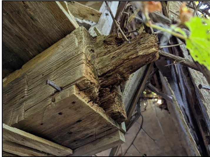
Photograph 6: Collapsed Floor on South Side of the House
