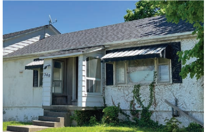
Asphalt roof shingles in good condition (ERA, 2025).
