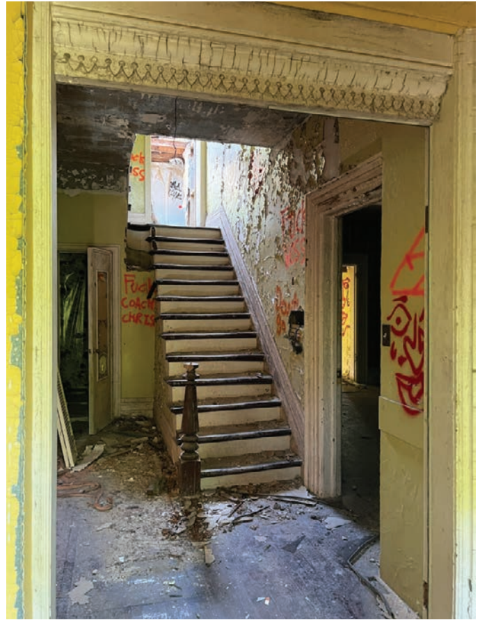
Looking into the front hall from the main entrance (ERA, 2025).
