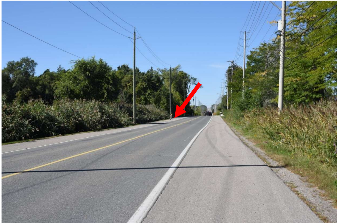
Exhibit 6-15: Stopping Sight Distance – South of Access (Looking Northbound from a point 105 m south of the access)
