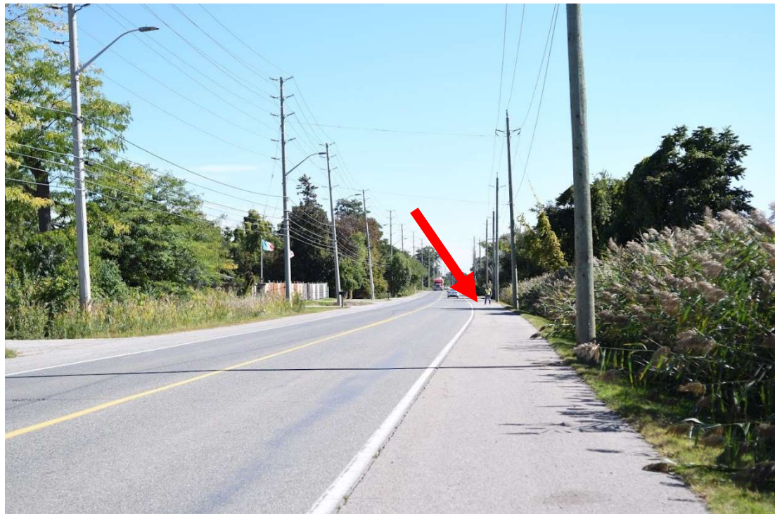
Exhibit 6-20: Stopping Sight Distance – North of Access (Looking Southbound from a point 105 m north of the access)
