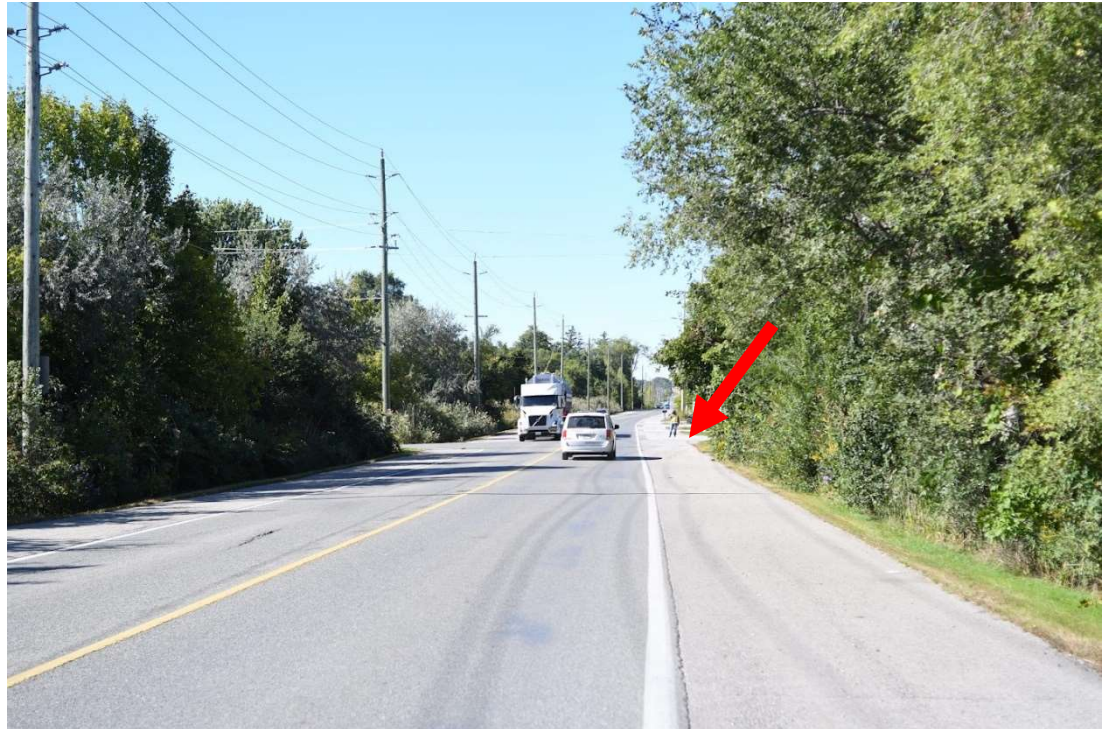
Exhibit 6-33: Stopping Sight Distance – South of Access (Looking Northbound from a point 105 m south of the access)
