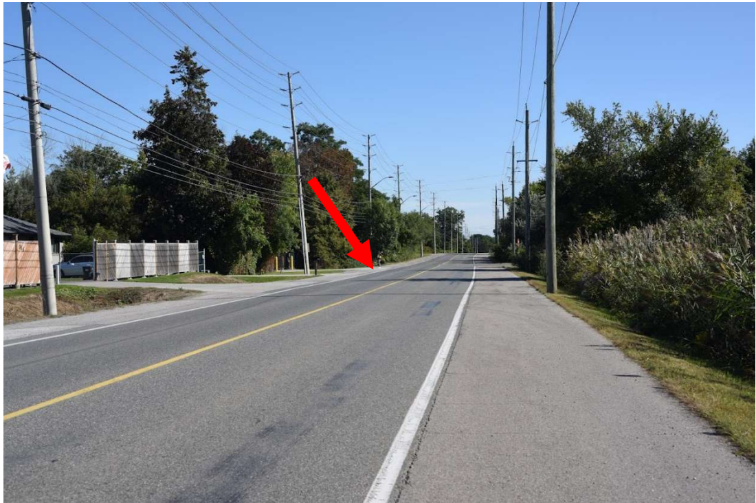
Exhibit 6-32: Stopping Sight Distance – North of Access (Looking Southbound from a point 105 m north of the access)
