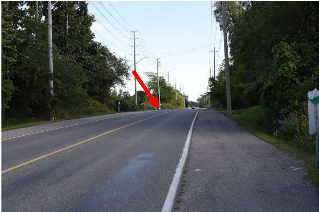
Exhibit 6-68: Stopping Sight Distance – North of Access (Looking Southbound from a point 105 m north of the access)
