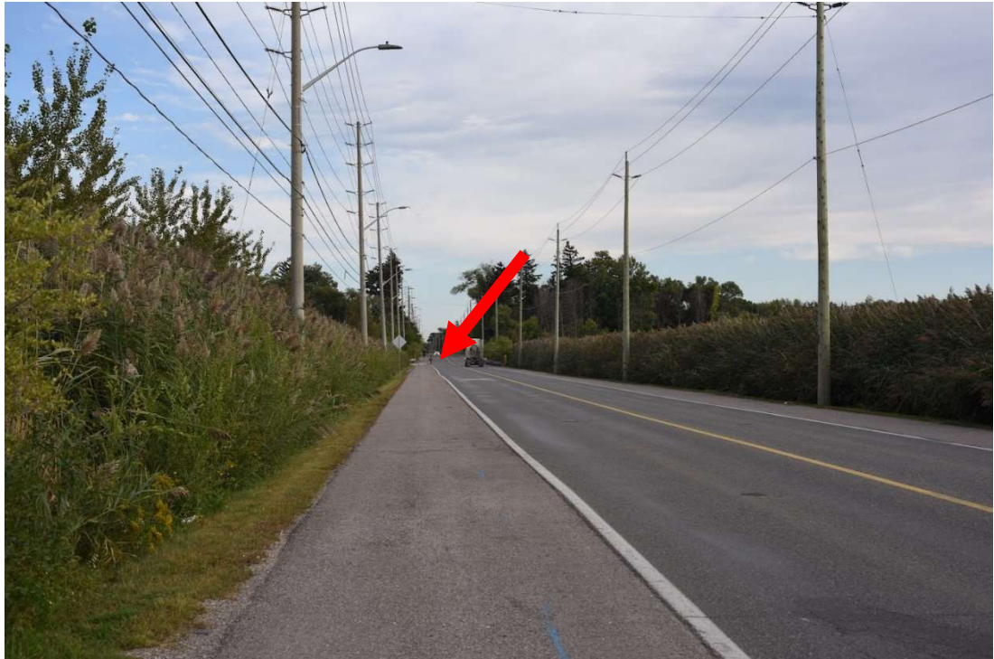
Exhibit 6-96: Departure Sight Distance – Looking South from the Access from a Position Approximately 1 m from the Edge of the Travelled Lane
