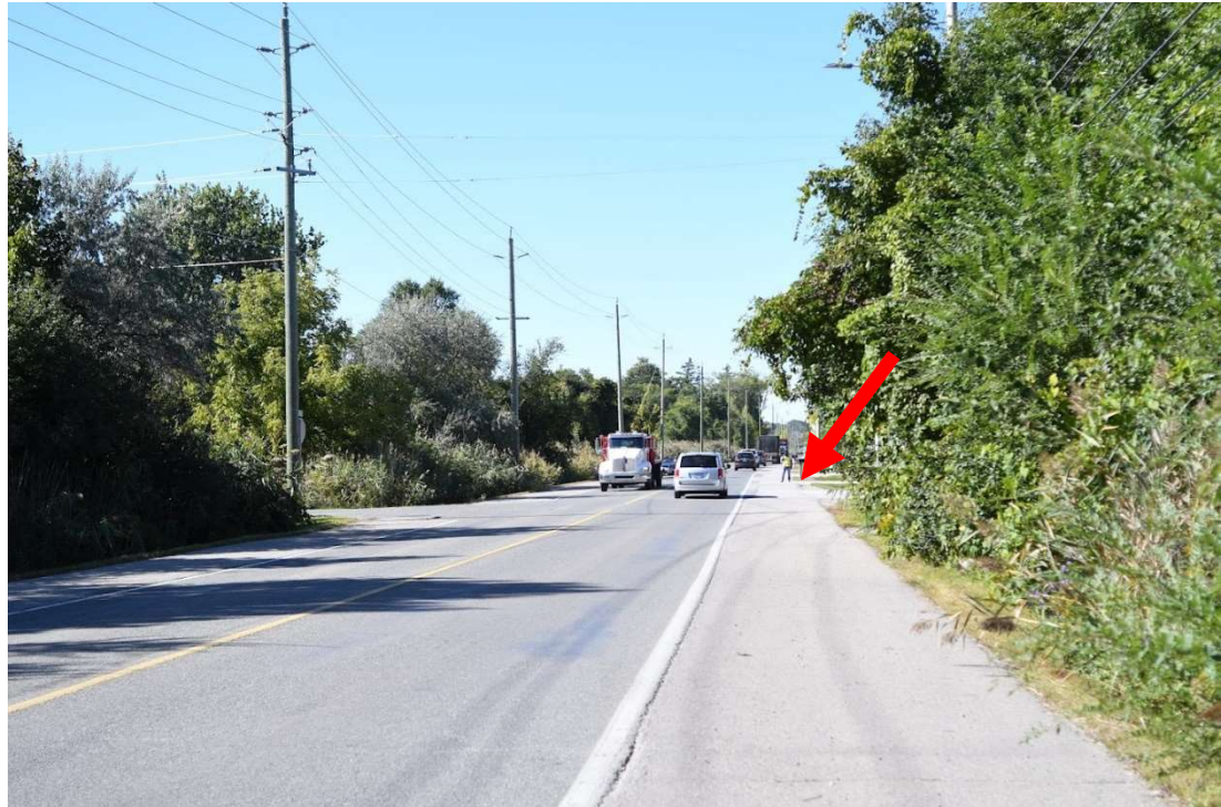
Exhibit 6-39: Stopping Sight Distance – South of Access (Looking Northbound from a point 105 m south of the access)
