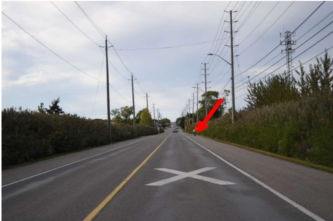
Exhibit 6-93: Stopping Sight Distance – South of Access (Looking Northbound from a point 105 m south of the access)
