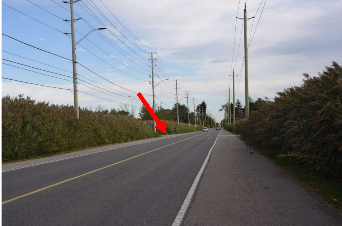
Exhibit 6-92: Stopping Sight Distance – North of Access (Looking Southbound from a point 105 m north of the access)
