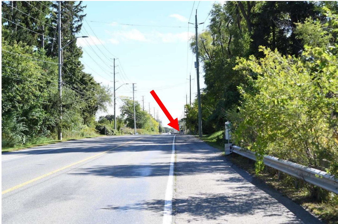
Exhibit 6-8: Stopping Sight Distance – North of Access (Looking Southbound from a point 105 m north of the access)
