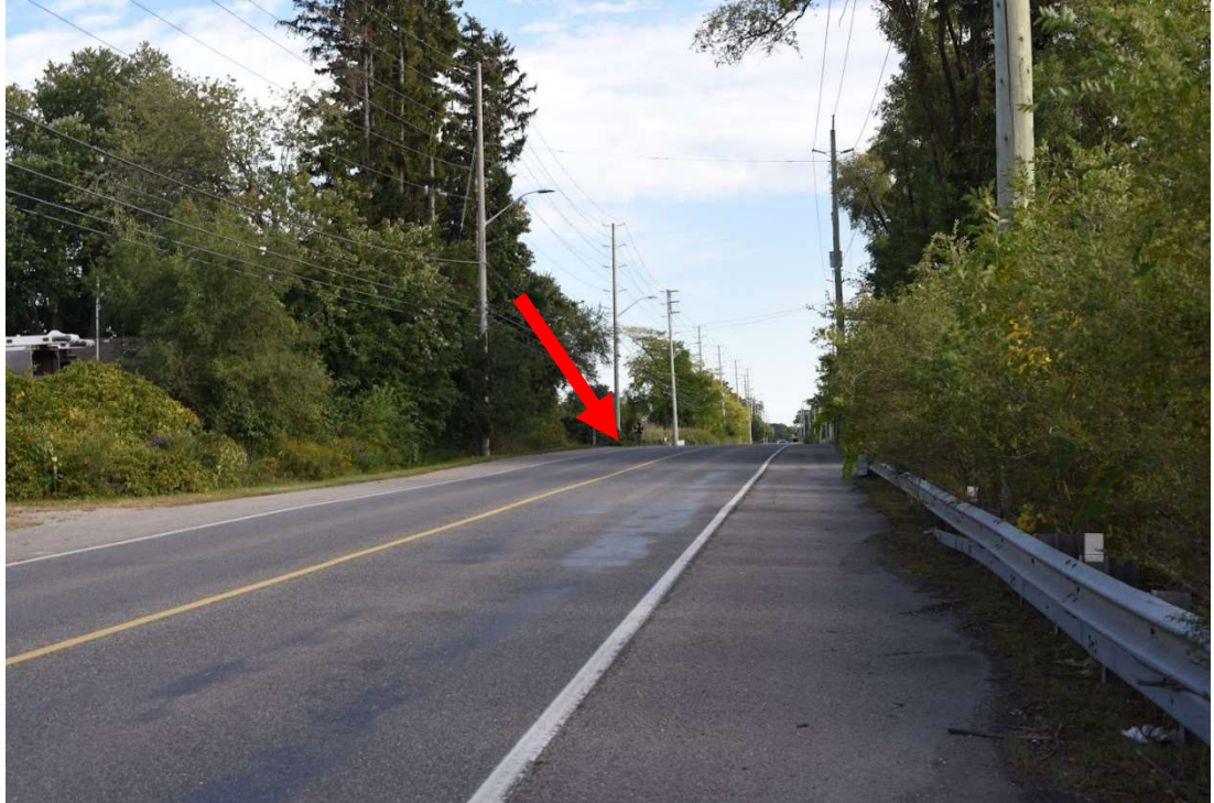
Exhibit 6-74: Stopping Sight Distance – North of Access (Looking Southbound from a point 105 m north of the access)
