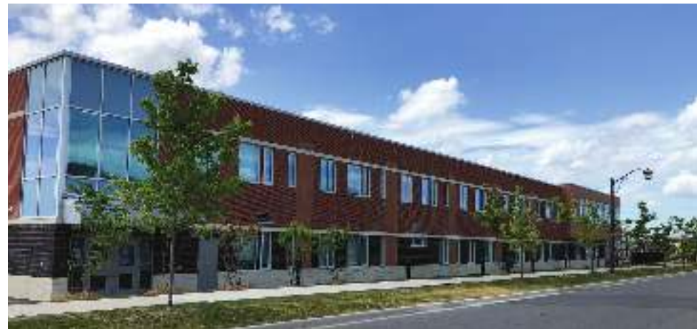
Fig. 6.6.6a - Examples of School Buildings
