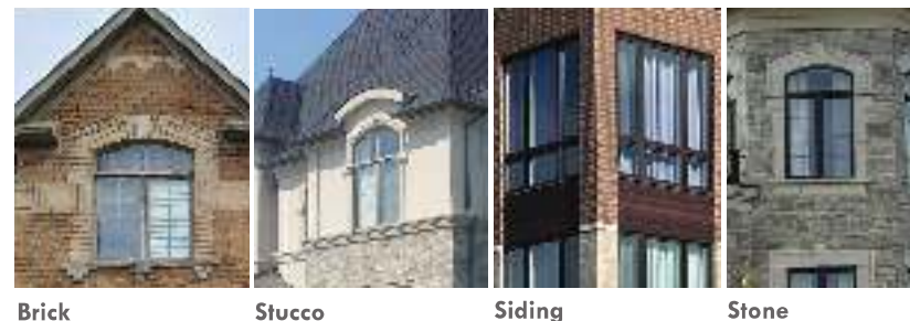
Fig. 7.4.2 - Examples of exterior main wall cladding materials
