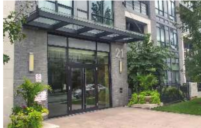
Fig. 6.6.5b - Main Entrances should be Designed as Focal Points for the Mid-Rise Buildings
