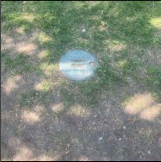
Image 11: Study Area showing in-ground water systems within the sports field.
