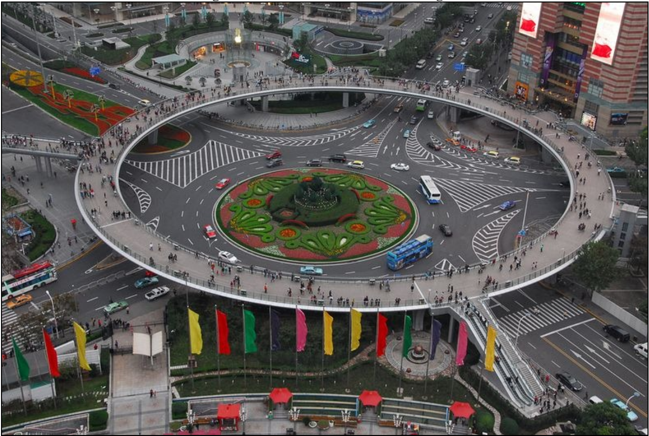
Figure 11-3: Elevated Pedestrian Bridge
