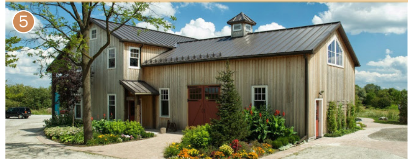
Fig. 2.2f - The Joshua Creek Heritage Art Centre, located northwest of the Phase 3 lands on Burnhamthorpe Road E
