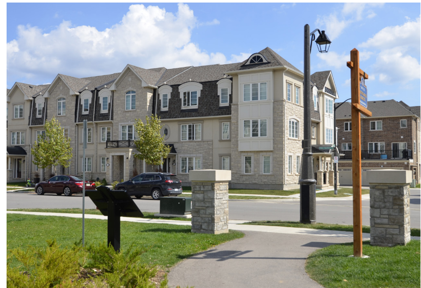
Figure 6.2b - Image example of 3-storey rear-lane townhouses facing an entrance into a neighbourhood park in North Oakville
