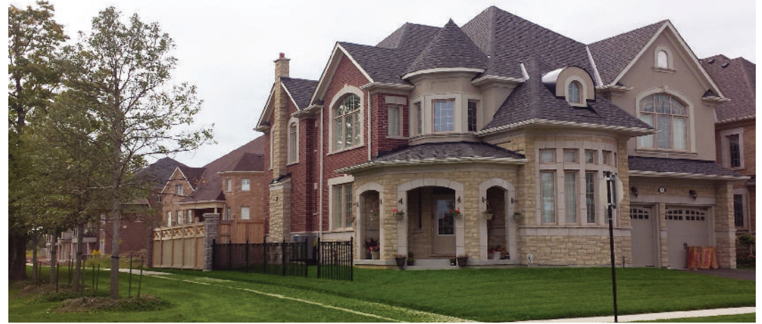
Fig. 7.8a - Example of a priority lot dwelling located at a corner that appropriately addresses both streets through architectural treatment (side-facing porch, wall articulation, windows, etc.)
