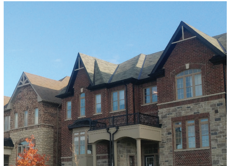
Traditional roof design
