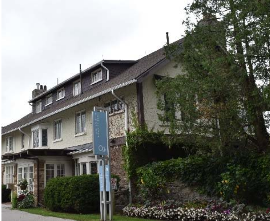
Figure 51: Gairloch Gallery north-east corner showing north wall of primary entry door 30 August 2018
