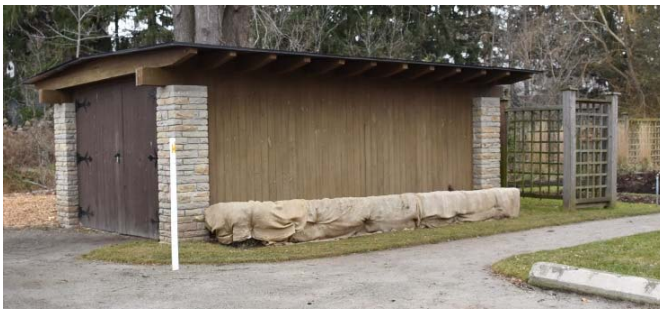
Figure 40: Equipment storage shed
