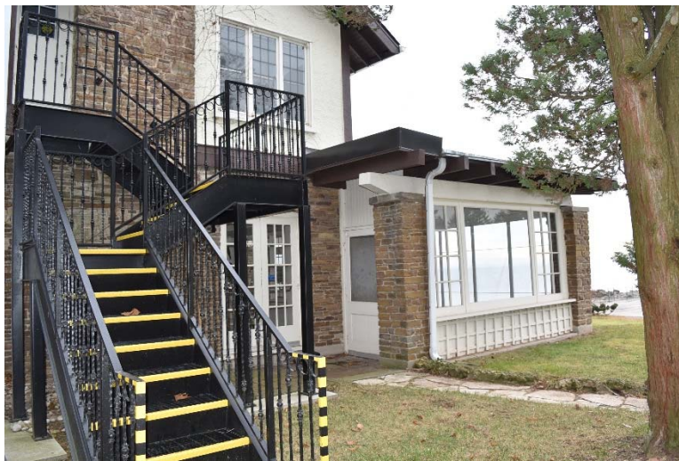
Figure 55: Gairloch Gallery, north façade. 20 December 2018
