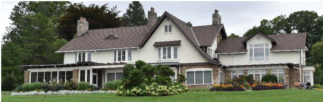
Figure 45: Gairloch Gallery west façade, 30 August 2018
