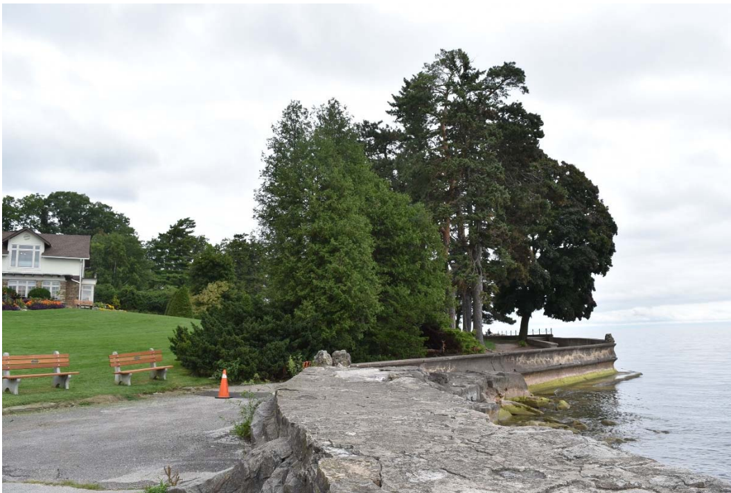
Figure 71: Stone and concave concrete retaining wall at Lake Ontario, looking east, 30 August 2018
