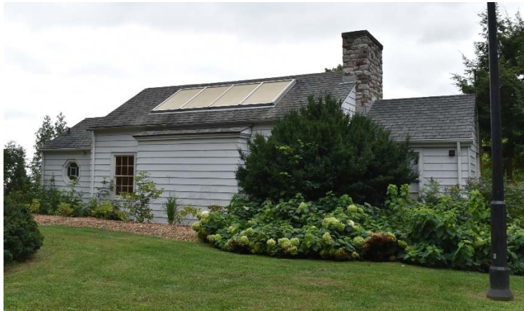
Figure 36: The studio, east façade, 3 October 2018
