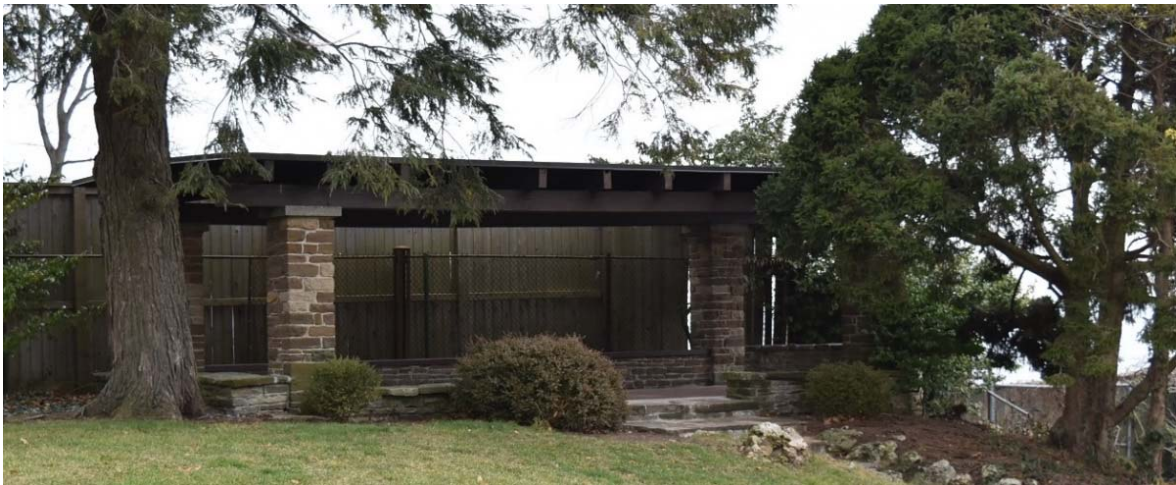
Figure 29: "The Look-Out", MacKendrick's teahouse. West façade, December 2018
