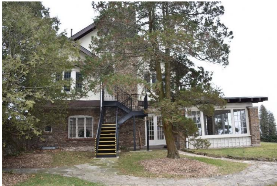
Figure 52: Gairloch Gallery, north façade. 20 December 2018
