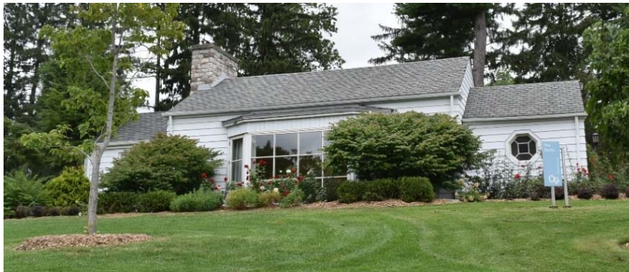
Figure 31: The Studio in Gairloch Gardens , west elevation, 30 August 2018
