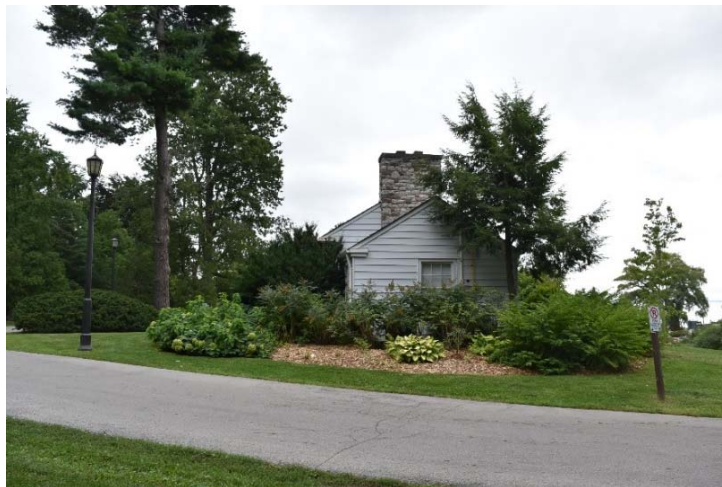
Figure 37: The studio, north façade, 3 October 2018
