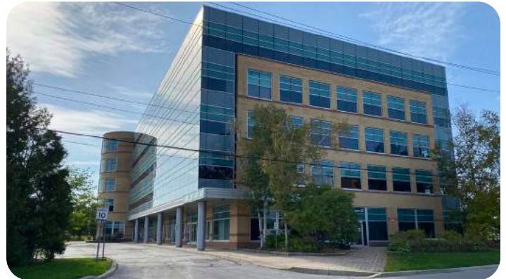
Office Building at 586 Argus Road
