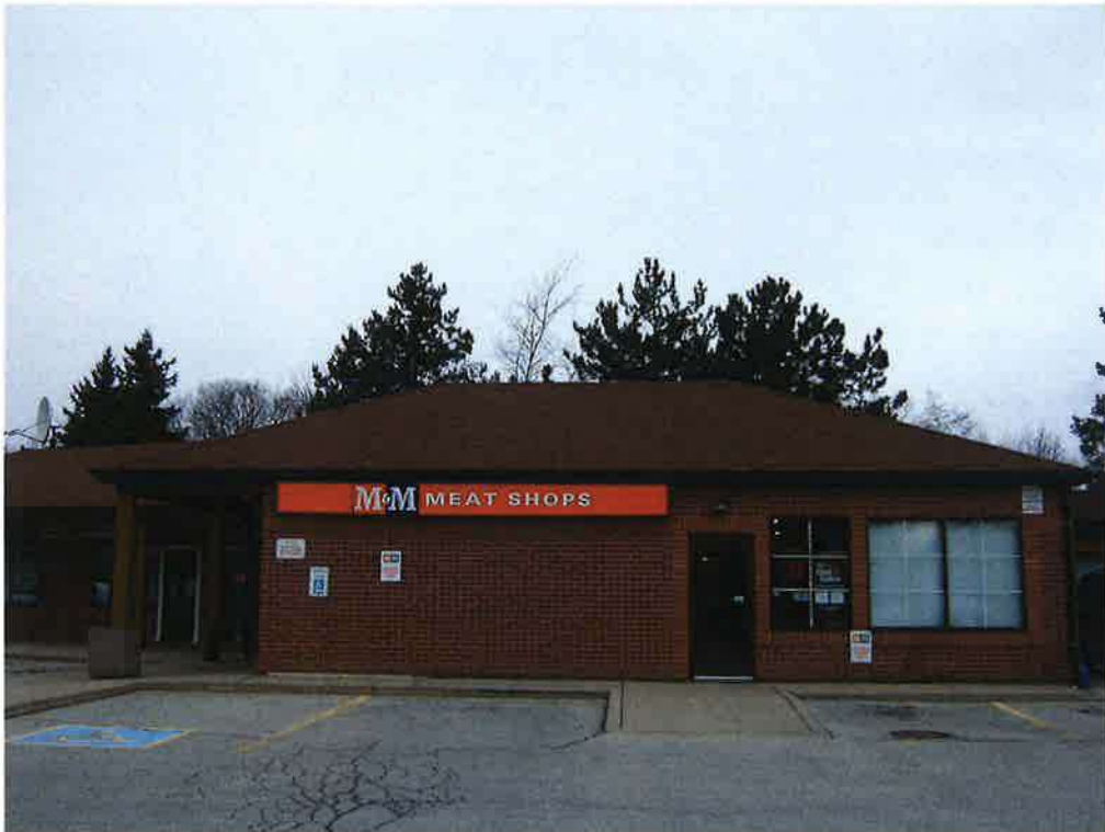
Northern portion of the subject site (Looking north)
