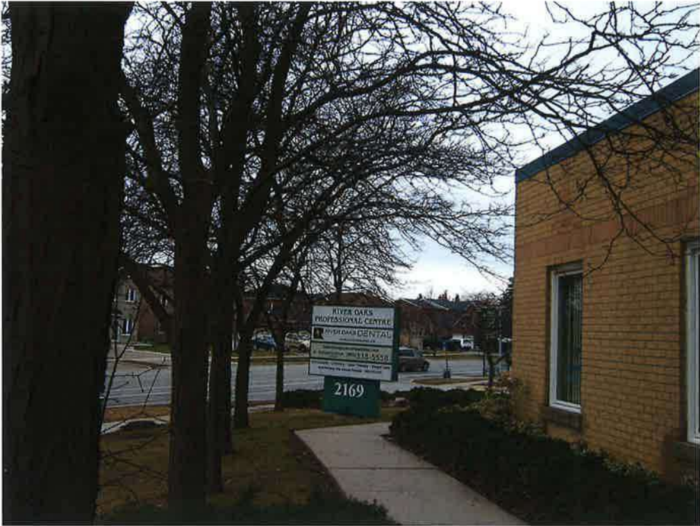
Southwestern portion of the subject site (Looking west)
