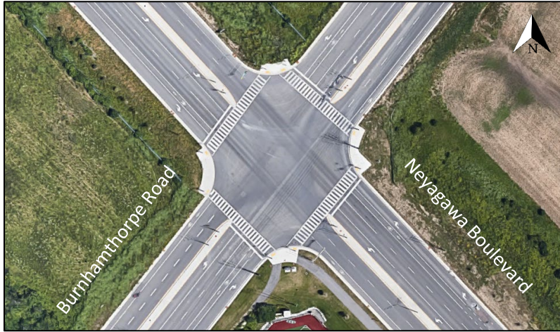
Figure 5: Intersection of Neyagawa Boulevard at Burnhamthorpe Road
