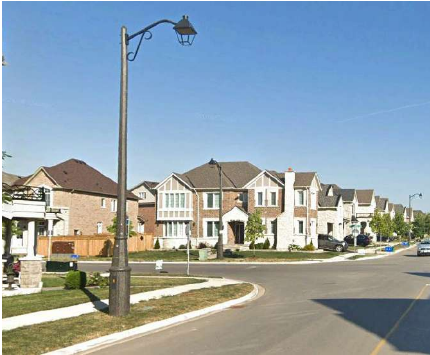
Fig. 6.2.1a - Street light poles and luminaires shall be consistent with the previous phases of The Preserve community
