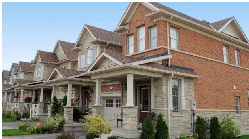
Fig. 6.3.2c - Image example of a range of building materials and colours that provide visual interest along the streetscape.
