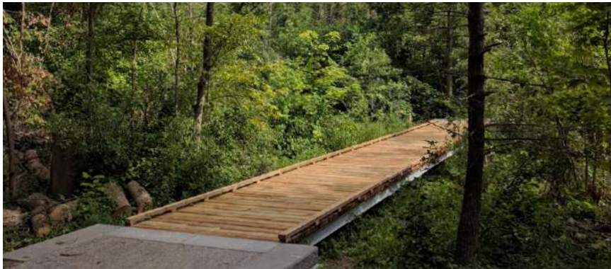
Fig. 6.1.4a - A Major Trail located south of the subject lands will be connected to the trail network proposed in Phase 4.
