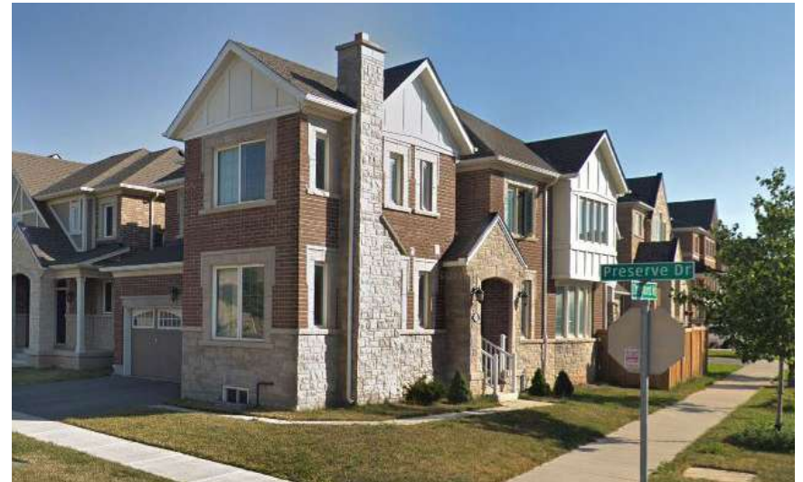
Fig. 6.4.1 - Image example of a corner lot dwelling in The Preserve that addresses both street frontages with the long elevation facing the flanking street.
