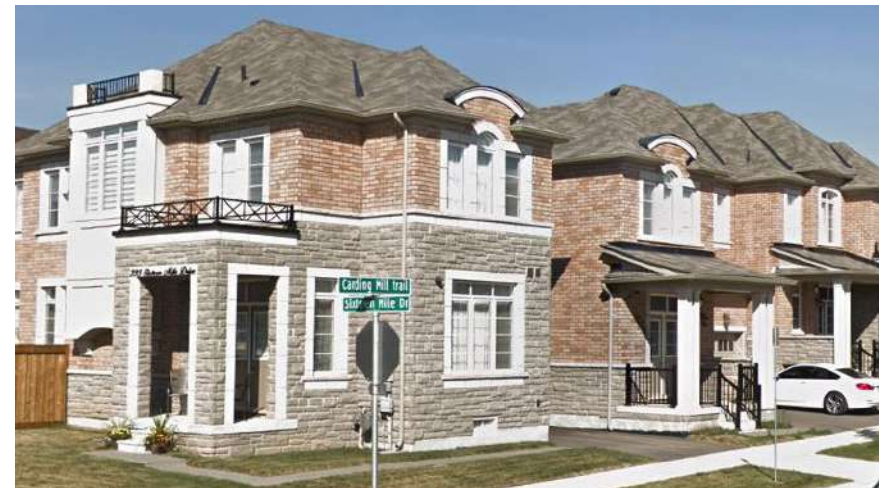
Fig. 6.2b - Existing street townhouses located on Carding Mill Trail, south of Phase 4
