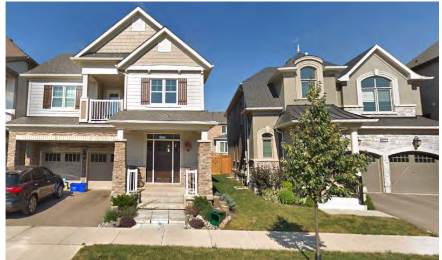
Fig. 6.3.2c - Image example a variety of single detached homes on Carding Mill Trail, south of Argo West Morrison.
