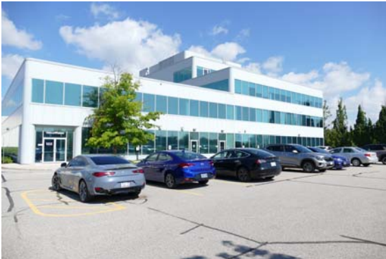
P4 - Partial view of the office building at 2360 Bristol Circle, facing north
