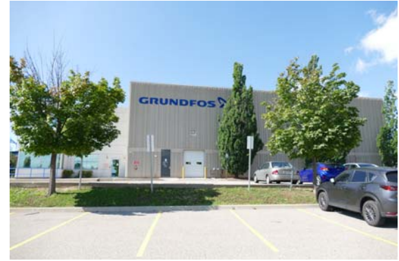
P9 - Neighboring property to the southwest
