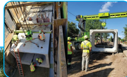
Storm sewer upsizing and superpipe storage
