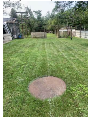
Picture 46: View of the covered well (no longer in use) at 1350 Bronte Road (July 21, 2021).
