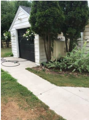
Picture 25: View of the AST at the side of 1316 Bronte Road (July 20, 2020).
