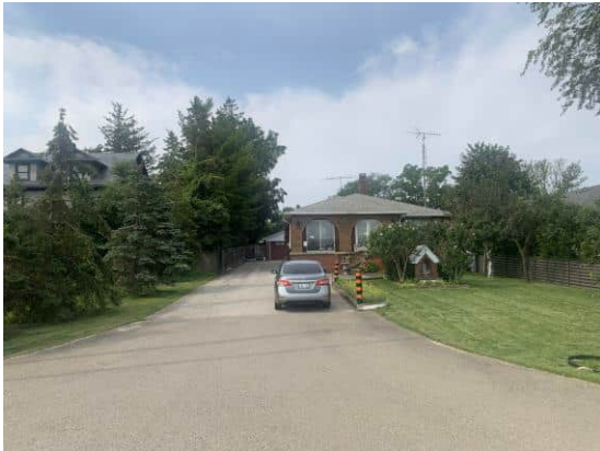
Picture 37: View of the residential building on the 1350 Bronte Road (July 21, 2021).
