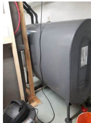
Picture 28: View of the AST at the basement of 1342 Bronte Road (July 31, 2020).
