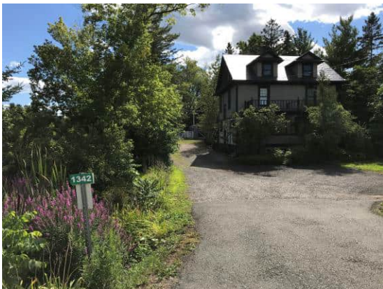
Picture 23: View of residential dwelling at 1342 Bronte Road (July 20, 2020).
