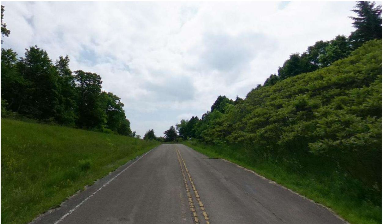
Photo 4: View of the trail to the south of Fourth Line connecting to the cemetery lands.
