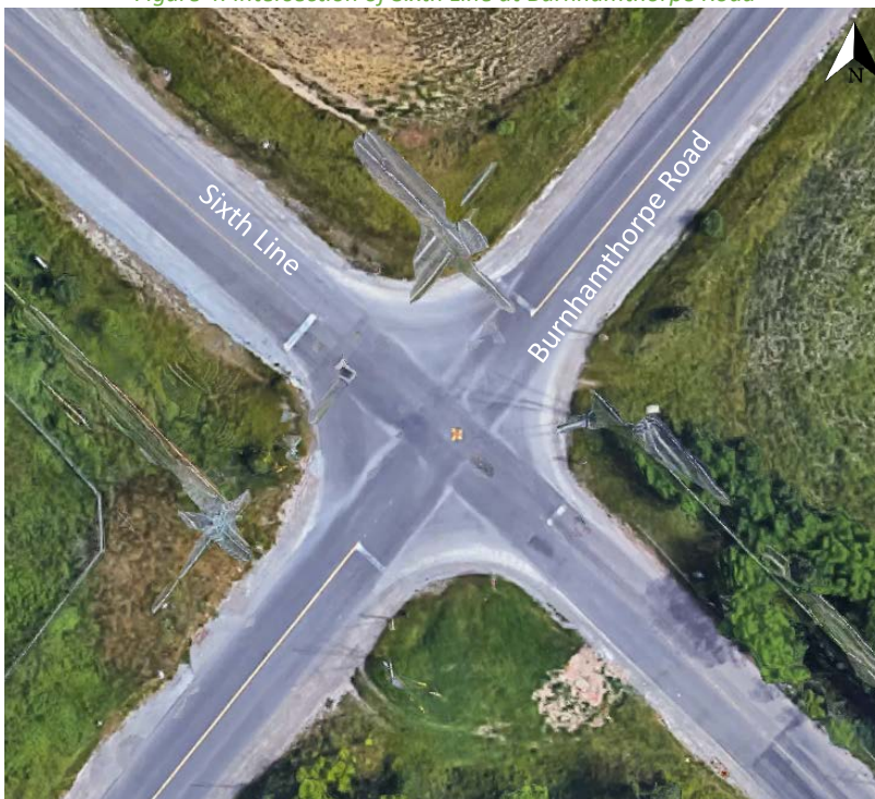
Figure 4: Intersection of Sixth Line at Burnhamthorpe Road
