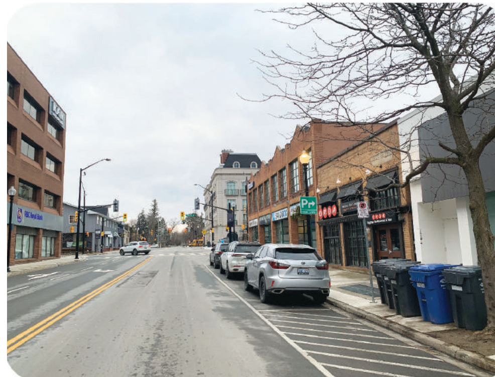
View along the Trafalgar Road looking north (south of Church Street)
