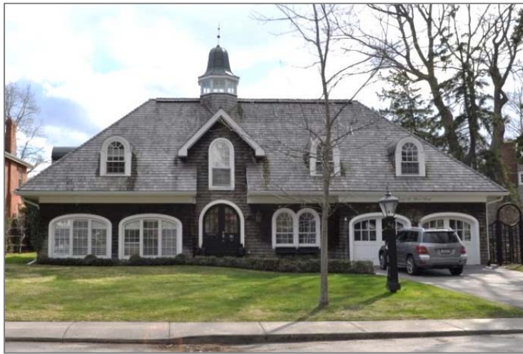
Figure 19: Integral garage at 46 First St
