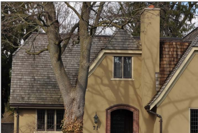
Figure 3: Cedar shingle roofing on 71 First St. (left); asphalt shingle roofing on 48 First St. (right).
