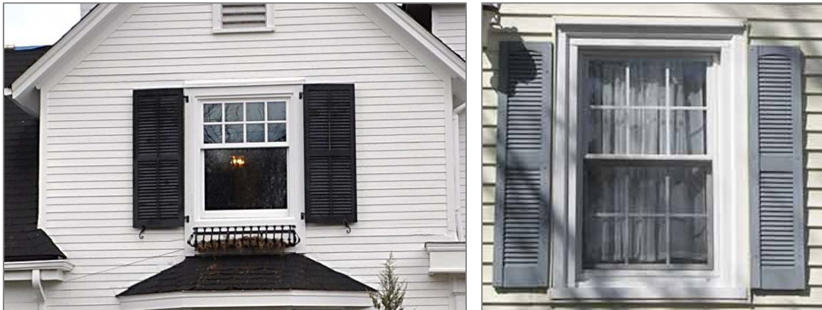
Figure 7: Appropriately-sized shutters on 66 Second St., (left); inappropriately small shutters on a building not located in the District (right) (source: http://www.oldhouseguy.com/shutters/ ).
