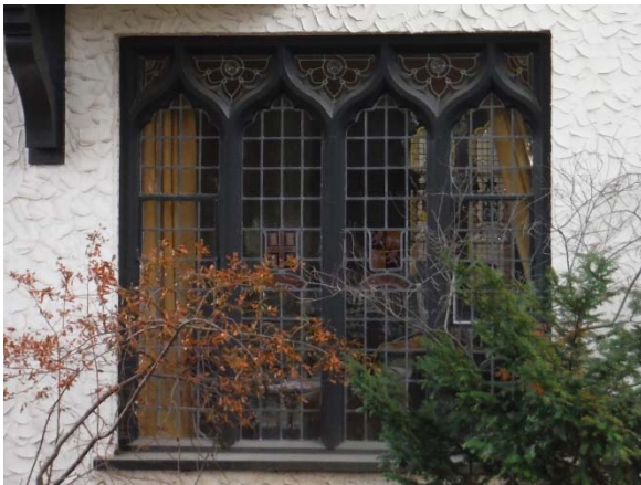
Figure 5: Leaded glass windows at 85 Second St. (left); wood windows with true divided lights at 75 Second St. (right).
