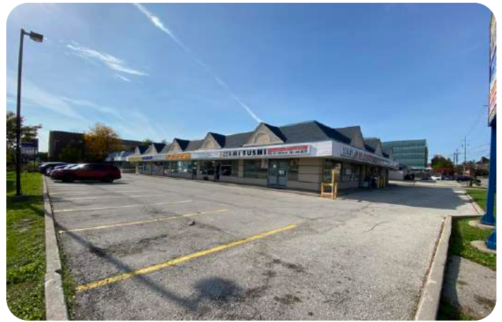
Commercial Plaza at (185-187 Cross Avenue )
