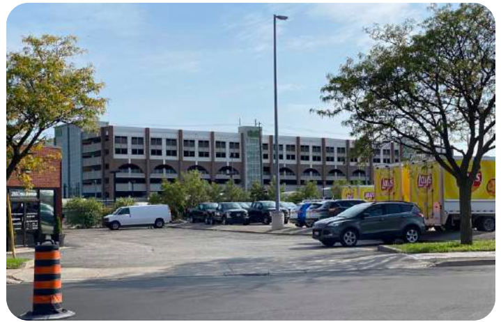
Ford Dealership parking area (foreground), GO Station Parking Structure (background)
