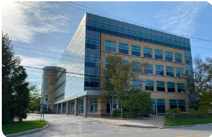
Office Building at 586 Argus Road
