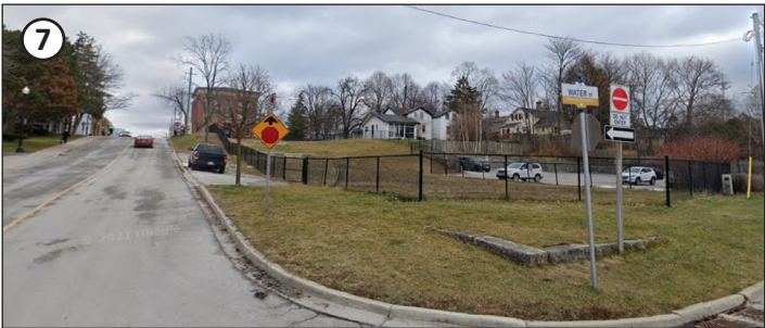
7 View of the site from Water Street
