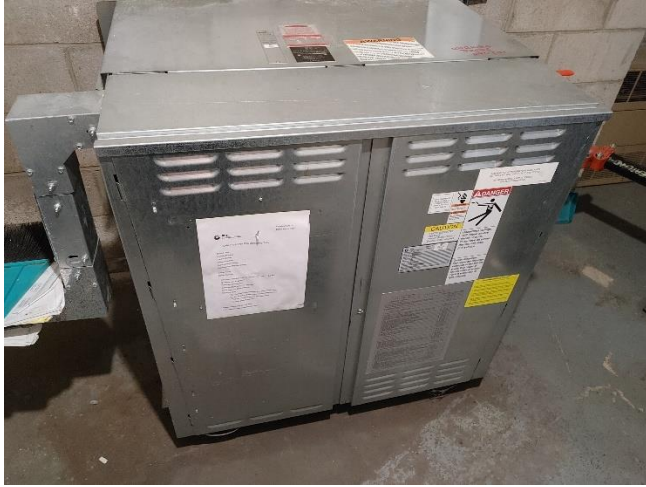
4- View of the oil tank for the hydraulic elevator in the lower-level elevator room
