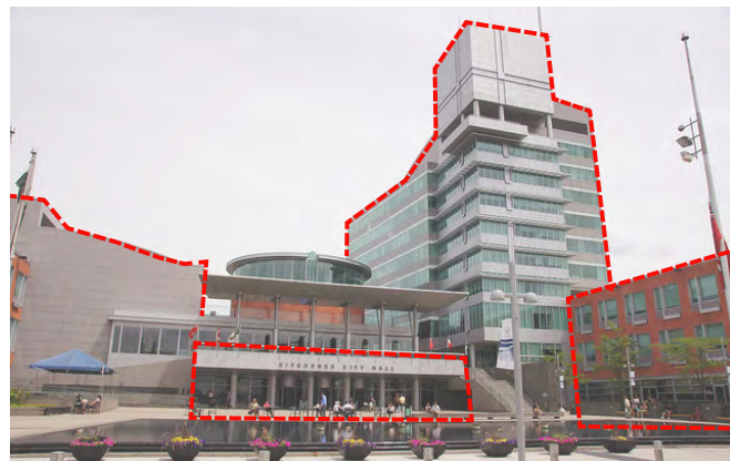
Kitchener City Hall, Kitchener, ON
