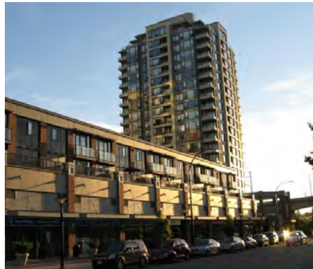
Tall building attached to low-rise residential, Vancouver, BC
