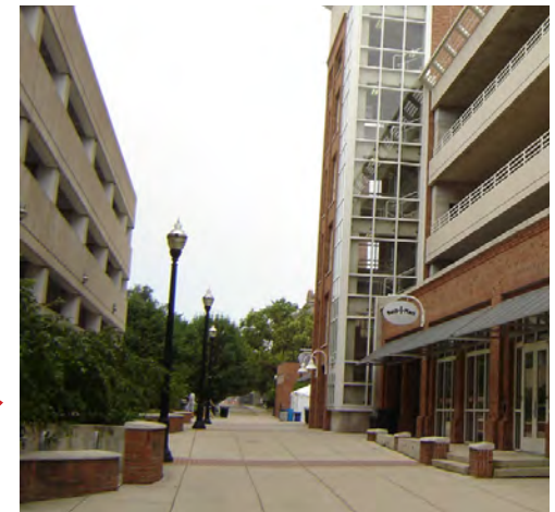
Ohio State Parking Garage, Columbus
