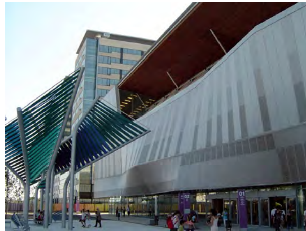
Barcelona International Convention Centre , Barcelona, Spain
