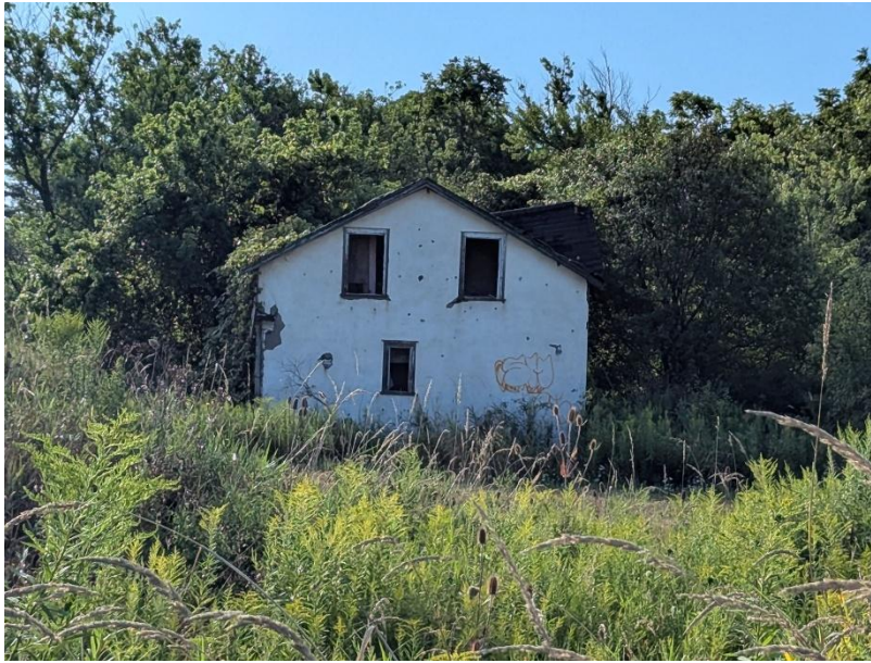
Image 1: View of house at 340 Burhamthorpe Road, in the centre of the study area.
