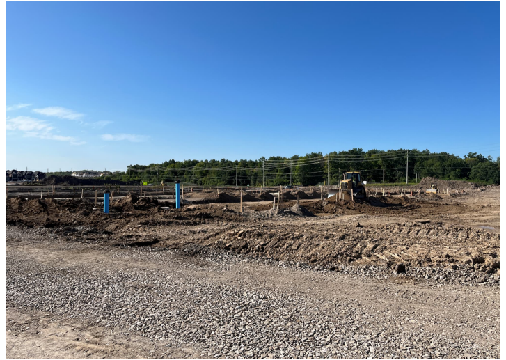
Photo 2: Southwestern portion of Site, facing southwest. Stockpile of topsoil observed in background.
