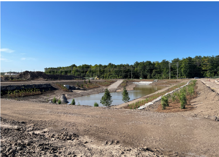
Photo 3: Stormwater management pond located in southwest portion of Site, facing southwest.
