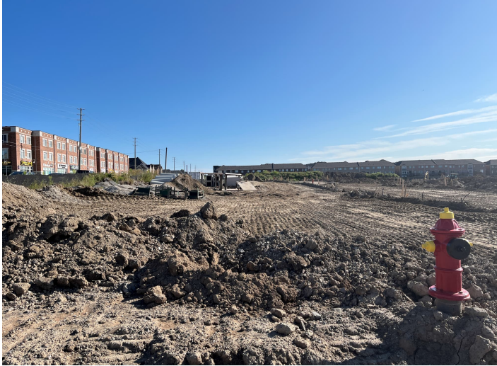
Photo 1: Northwestern portion of Site, facing northeast.
