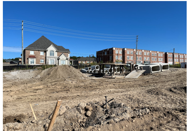
Photo 4: Storage of concrete pipes, trench boxes, catch basins along northwestern edge of Site, facing north. Pile of imported granular observed.
