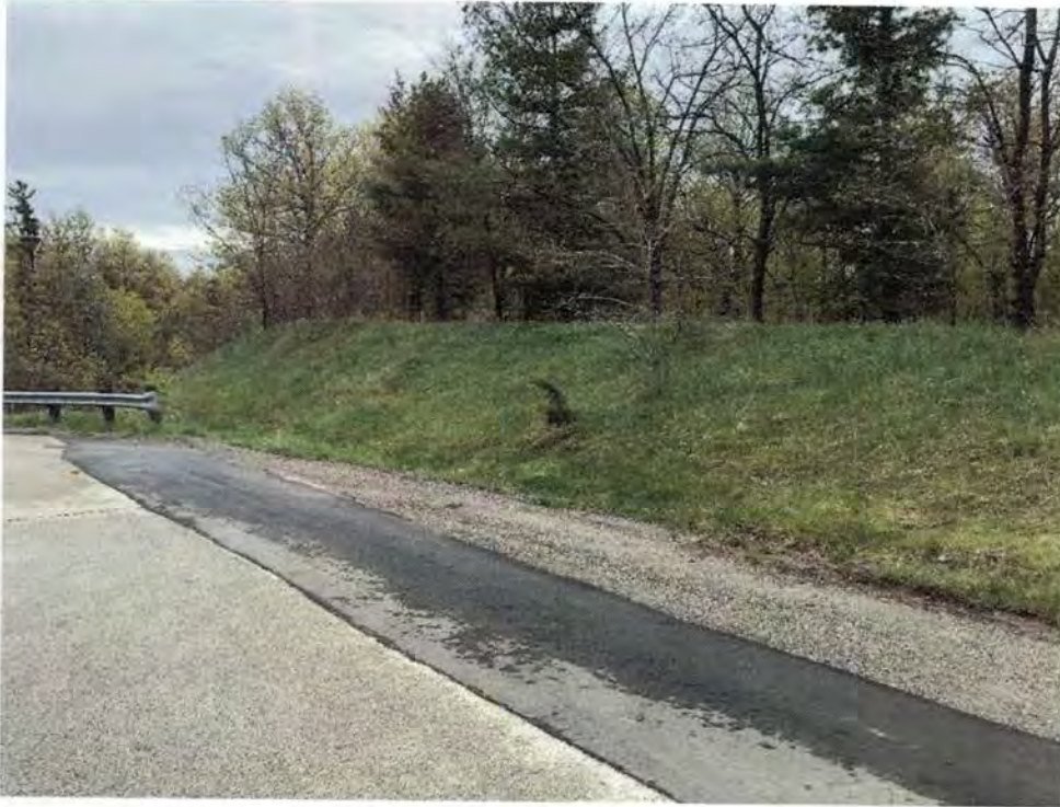
West Slope – Looking south, Cross Section C
