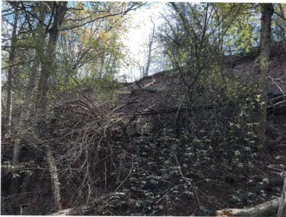
Sixteen Mile Creek Slope – Slope overburden erosion, looking West
