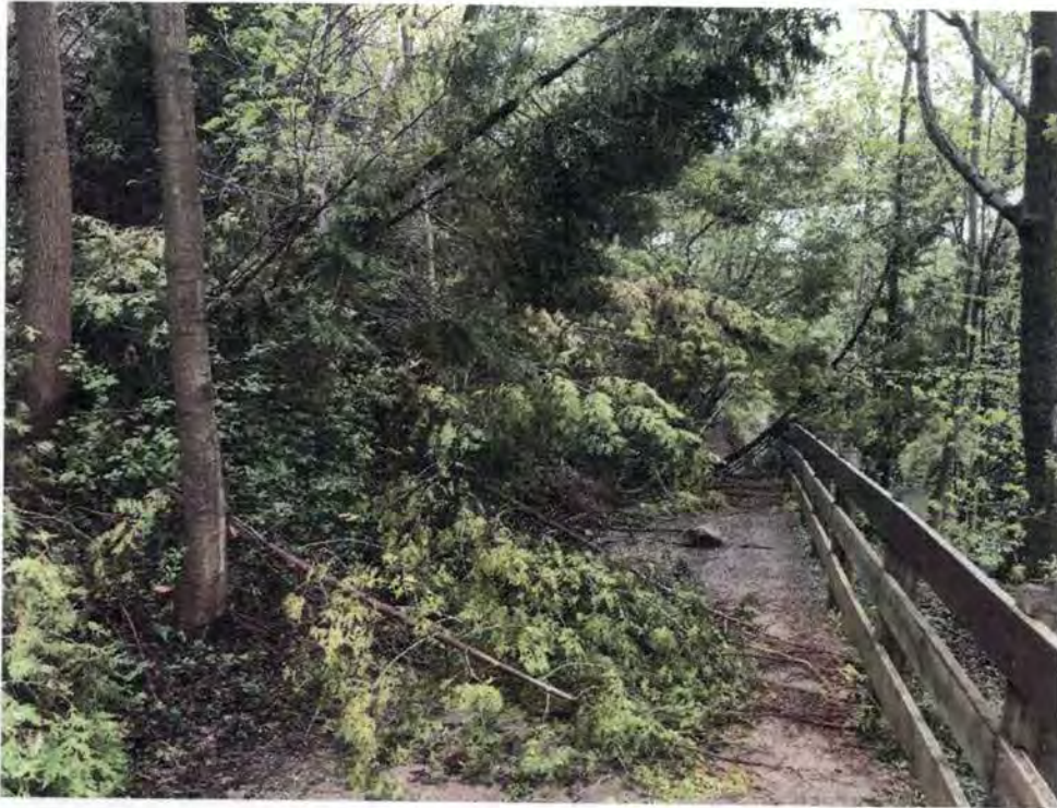
Sixteen Mile Creek Slope – Looking Southwest, slope overburden erosion impeding path, Cross Section B
