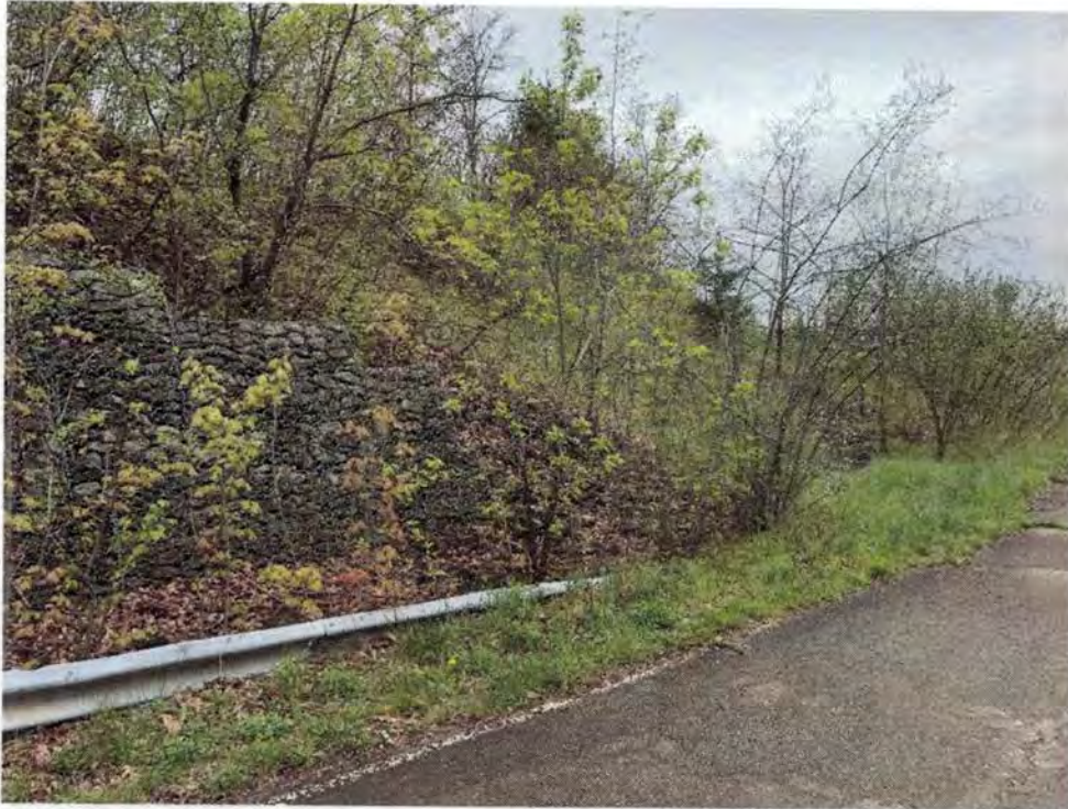
West Slope – Looking North, Gabion Retaining Wall
