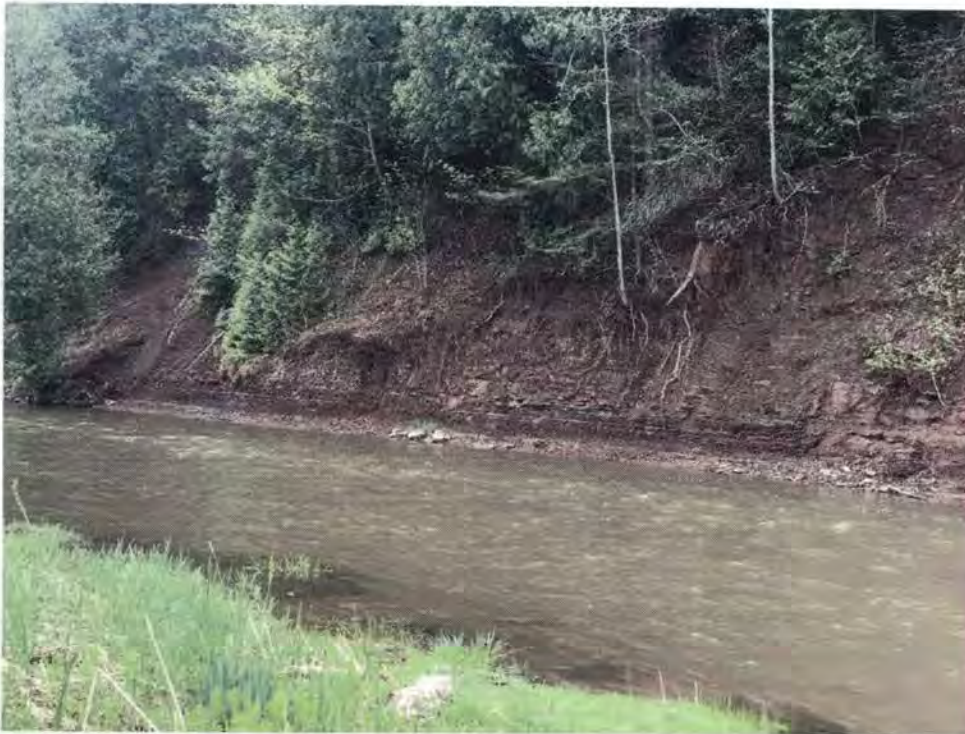
Sixteen Mile Creek Slope – Toe of slope, looking southwest, Cross Section C
