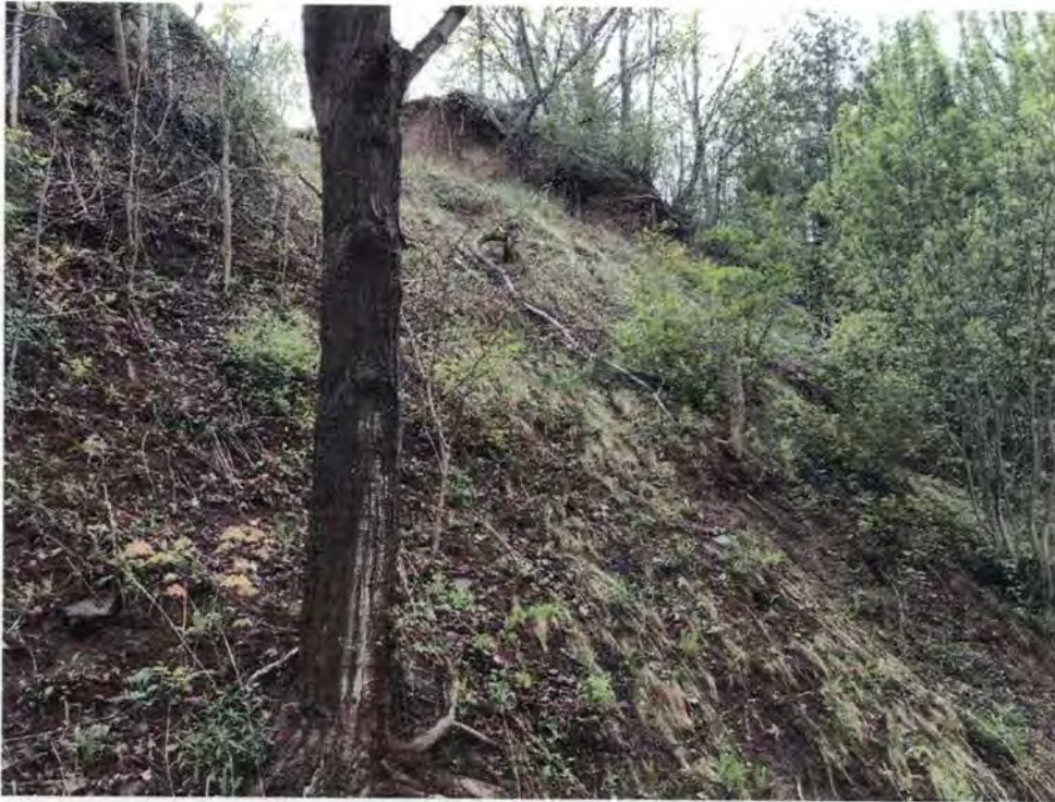
Sixteen Mile Creek Slope – Looking Northwest, Cross Section C
