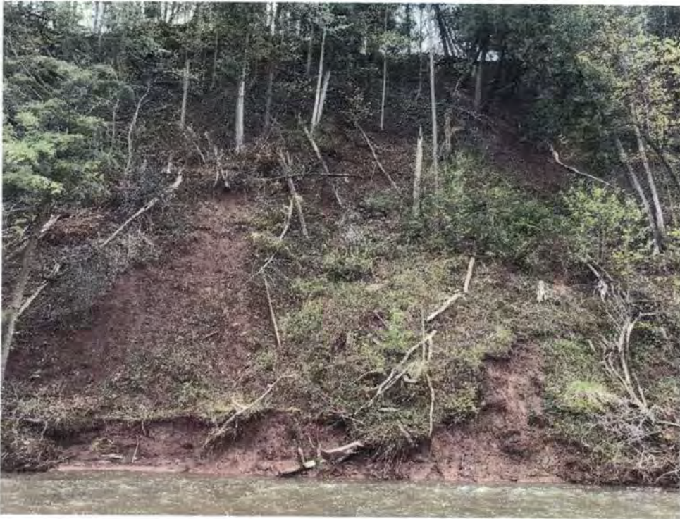
Sixteen Mile Creek Slope – Toe of slope, looking West
