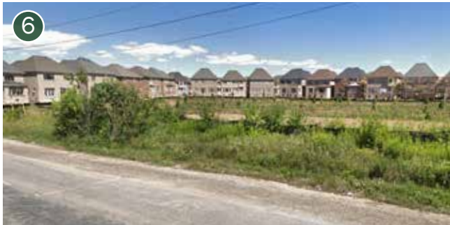
Existing single detached houses under construction backing onto NHS channel along east side of Sixth Line, south east of the Argo West Morrison subject lands.
