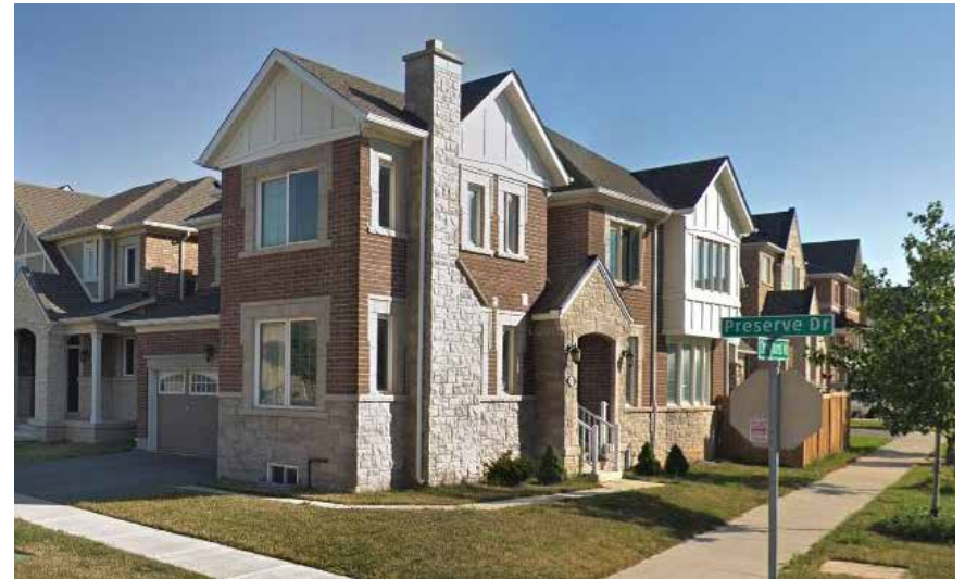
Fig. 6.4.1 - Image example of a corner lot dwelling in the adjacent community that addresses both street frontages with the long elevation facing the flanking street.
