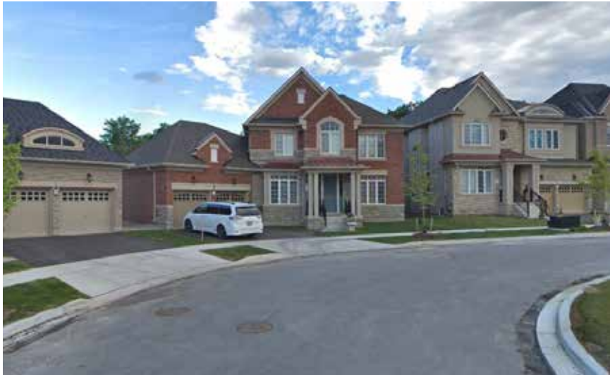
Fig. 6.4.2 - Image example of a view terminus dwelling in the adjacent community, with a prominent architectural entry at the terminus view
