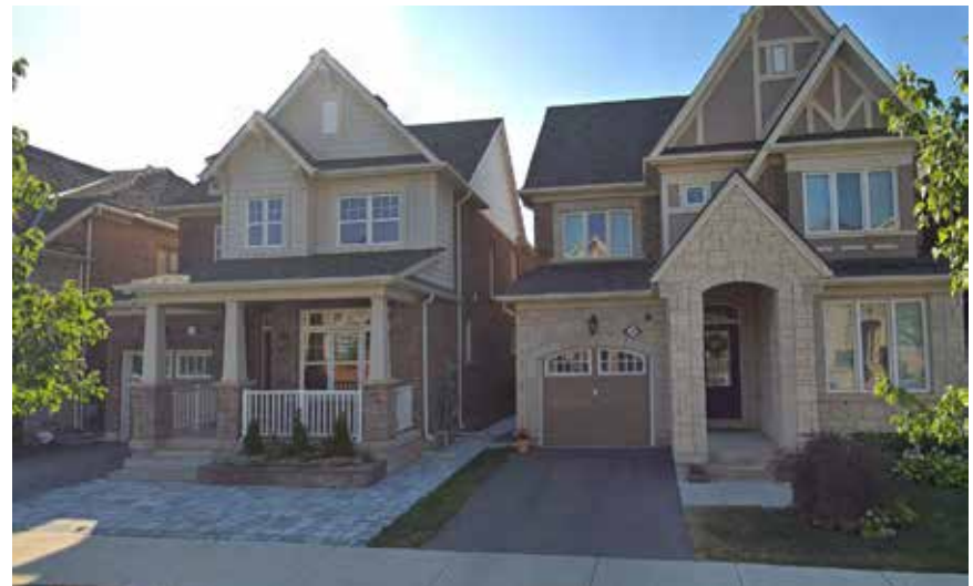
Fig. 6.3.2d - Image example of attached garages integrated into the main massing of the dwelling, behind the porch projection.
