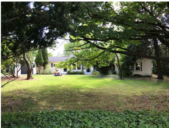
Picture 21: View of residential dwelling at 1316 Bronte Road (July 20, 2020).
