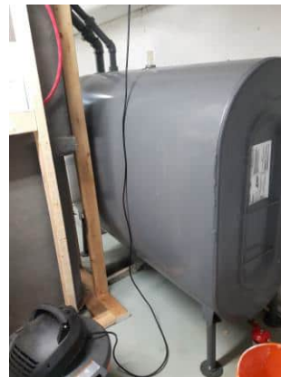
Picture 28: View of the AST at the basement of 1342 Bronte Road (July 31, 2020).
