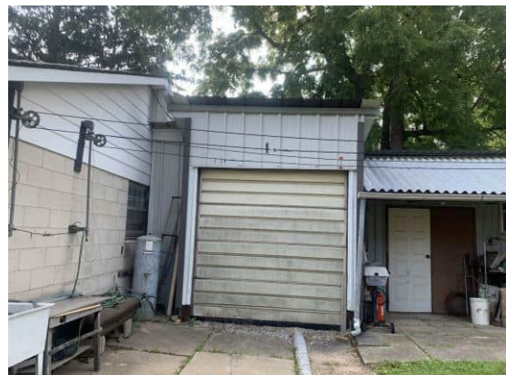
Picture 42: View of the garage at 1350 Bronte Road (July 21, 2021).
