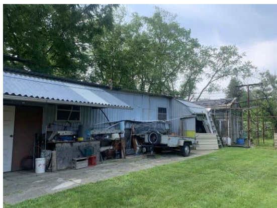
Picture 43: View of the work shed at 1350 Bronte Road (July 21, 2021).
