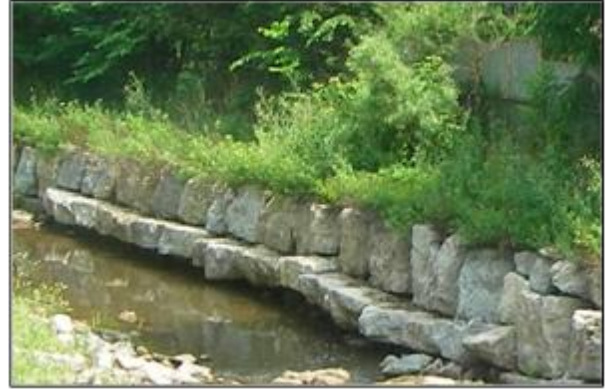
Armour Stone Wall with Brush Layer Concept
