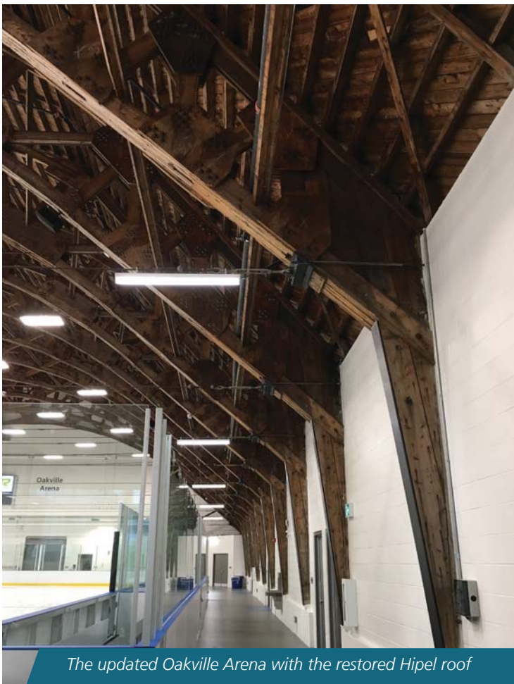
Roof extension added to accommodate a NHL-size rink – the new wood ceiling is lighter to differentiate the old from the new
