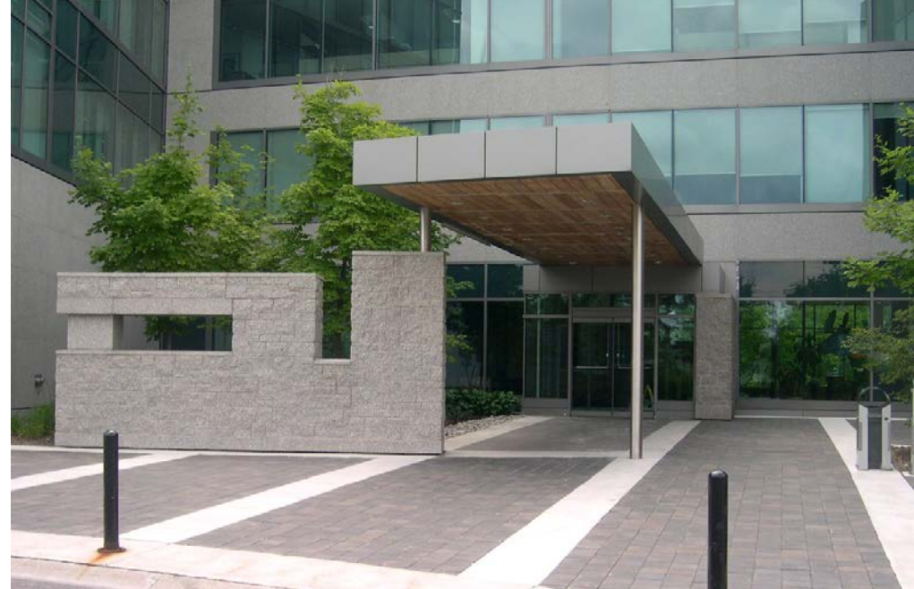
Fig 6.3.2a - Main entrances shall be designed with emphasis, using high-quality exterior cladding materials
