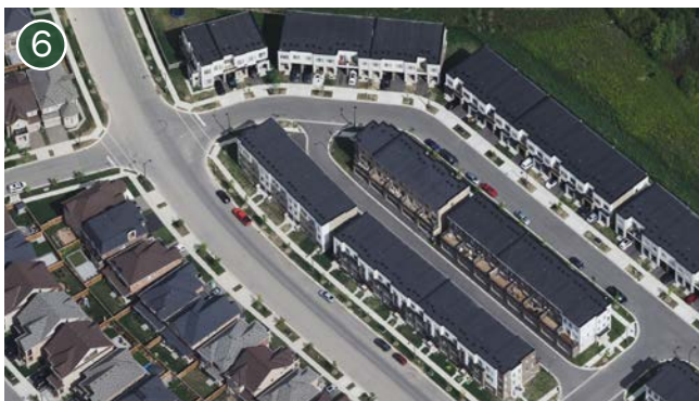
Bird's eye view of newly constructed rear lane townhomes on Ernest Appelbe Boulevard, south-east of Sixth Oak
