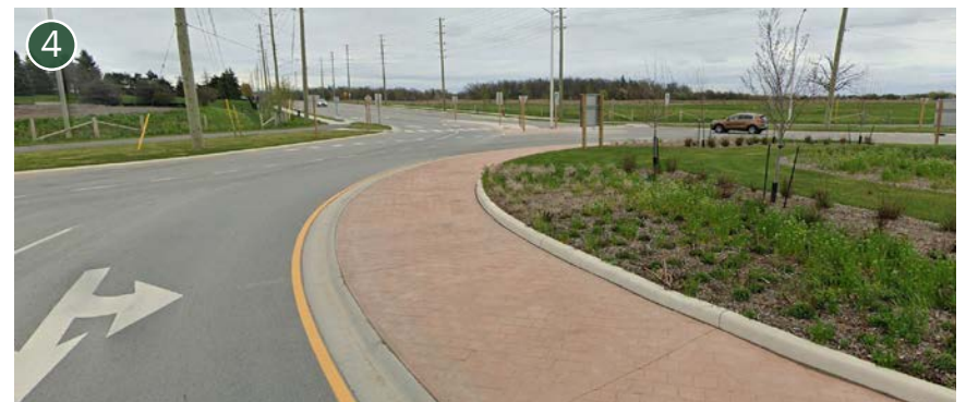
Newly constructed roundabout at William Halton Parkway and Sixth Line, looking south-west toward the Sixth Oak subject lands
