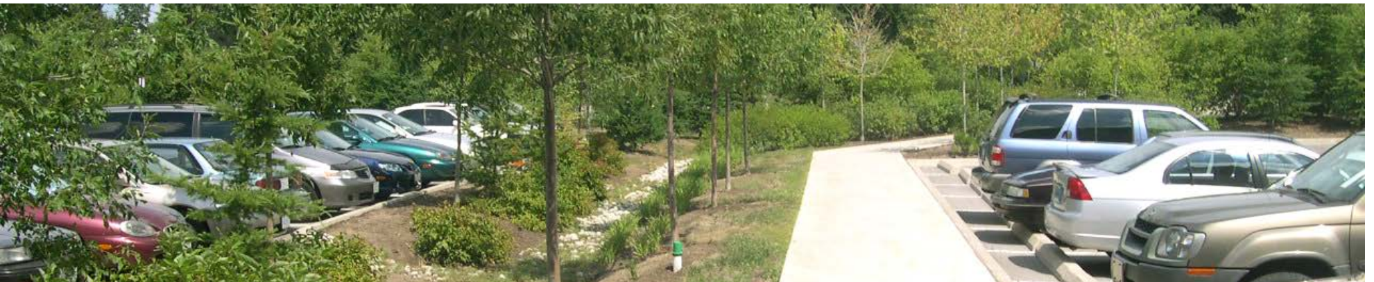
Fig 6.4 - Where feasible, integrate bio-retention swales as an effective technique for managing stormwater within parking lots
