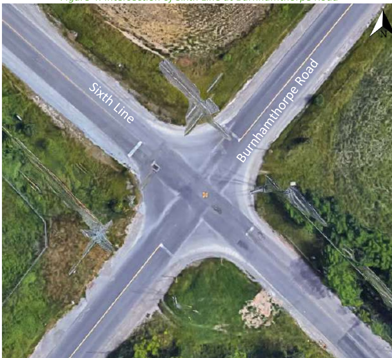
Figure 4: Intersection of Sixth Line at Burnhamthorpe Road
