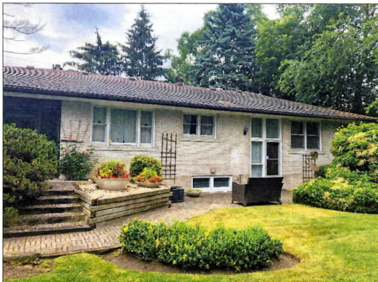
Photograph 4 – Site Building (northwest side).
