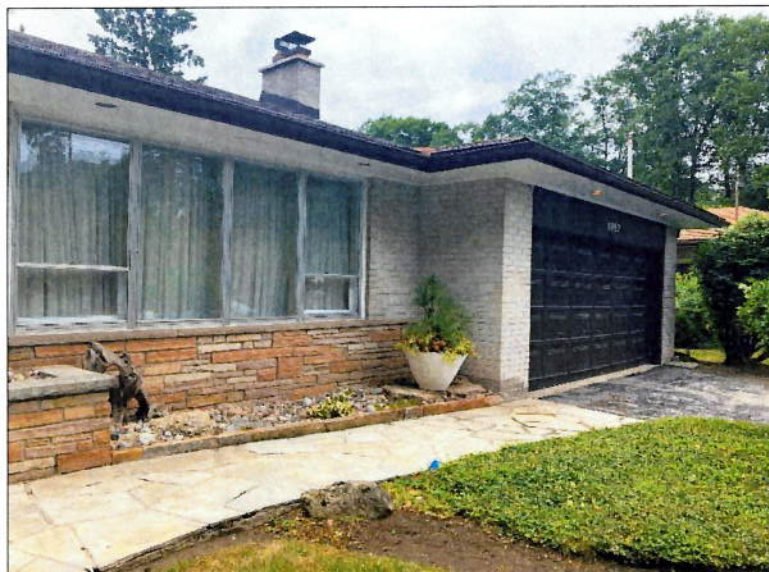
Photograph 2 – Site Building (southeast side).
