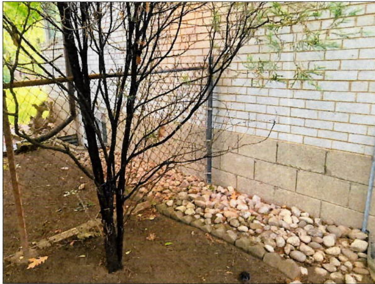
Photograph 3 – Site Building (southwest side).
