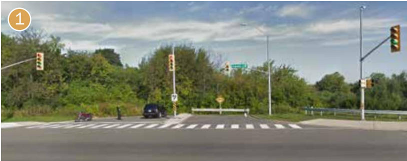
Fig. 2.2b - View facing north from Dundas Street E and Meadowridge Drive, which extends into the lands to the east of Phase 4
