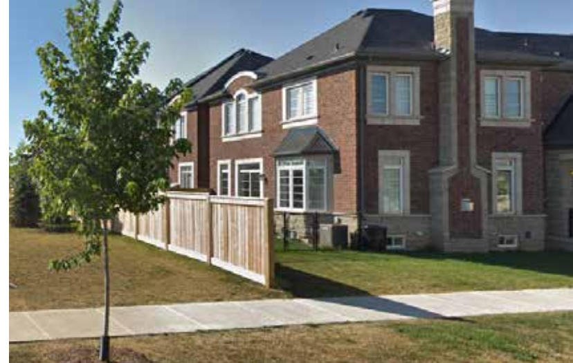
Fig. 6.4.3 - Image example of an upgraded side architecture dwelling with wall articulation, ample fenestration and interesting roof line.
